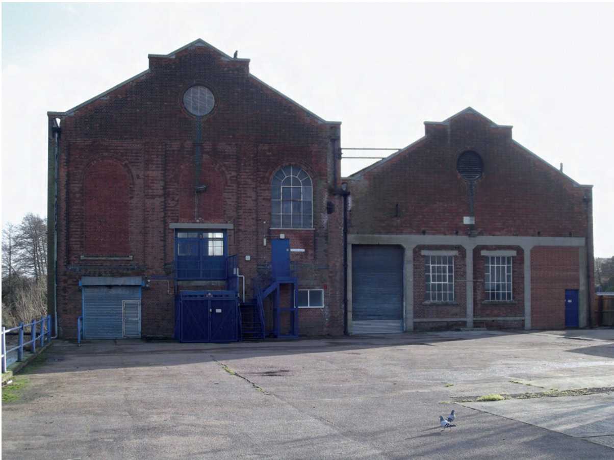
PLATE 11: Power House, Factory Lane West, Halstead, built in 1922 to provide power to the Courtauld's weaving factory. (Tony Crosby)
