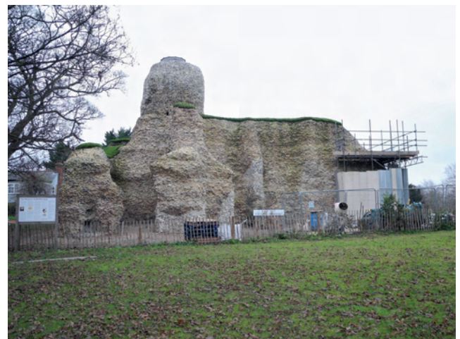
FIGURE 2: The south side of the keep in December 2016 showing the remains of the forebuilding. The turret is a semaphore tower built in the late 18th century
