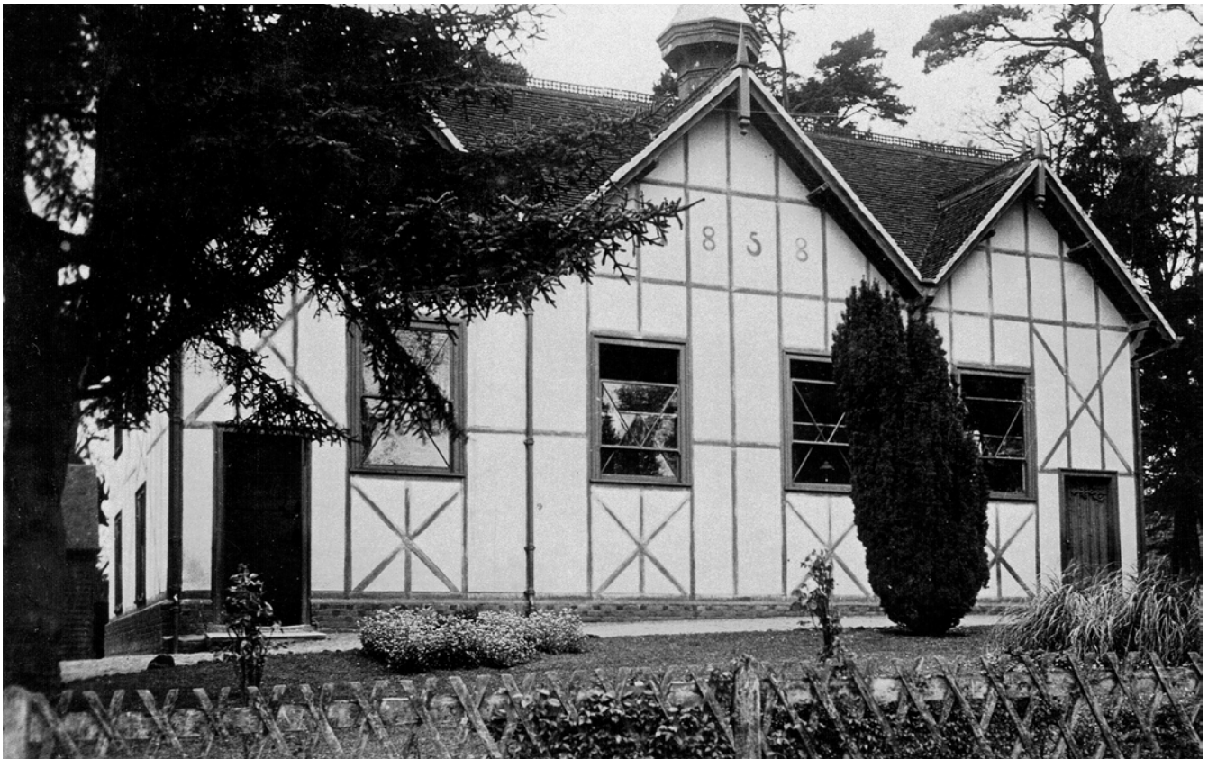
PLATE 9: Lecture Hall (now Primary School), The Street, Gosfield, built in 1858 by Samuel Courtauld. (Adrian Corder-Birch Collection)
