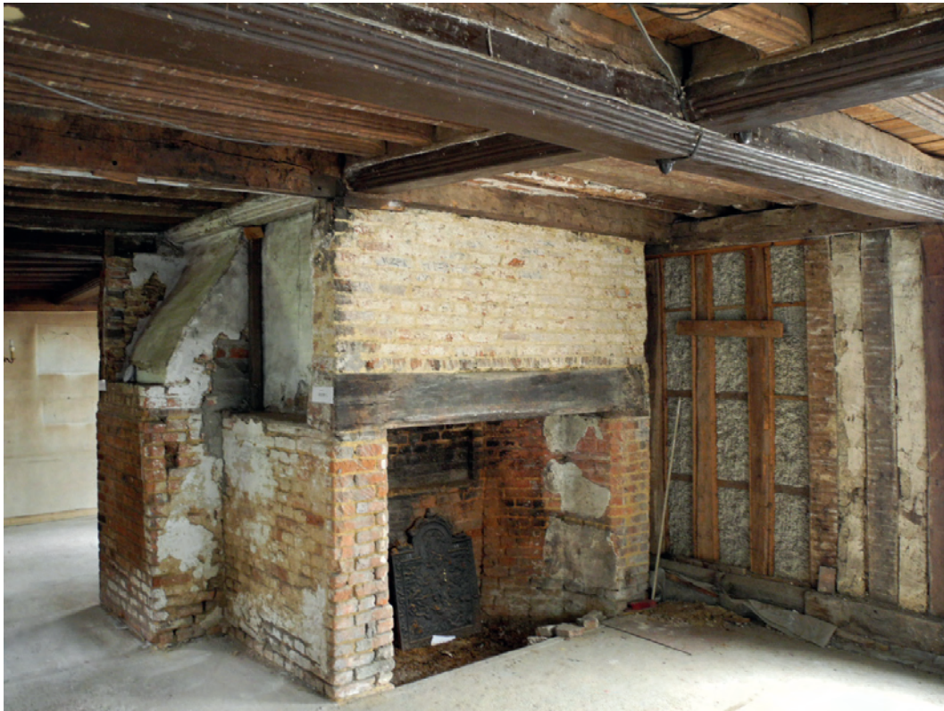
FIGURE 5: The fireplace seen from the south
