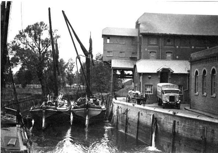
Barges unloading, note the grain sucker, the pipe extending from the lucam and dropping down to the right hand barge.
