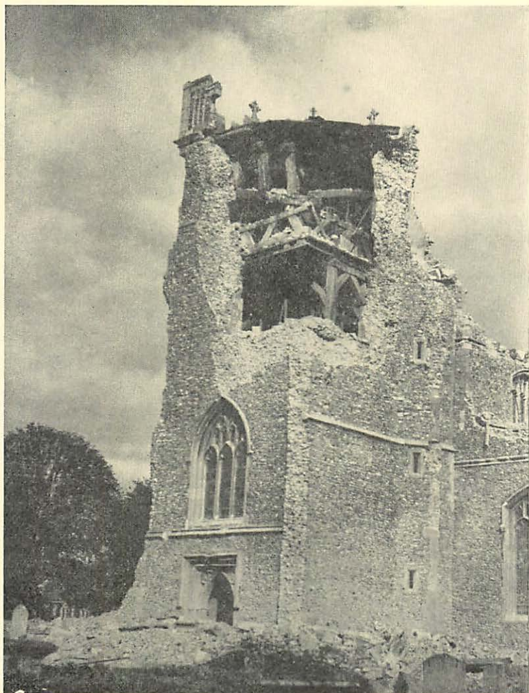
COGGESHALL CHURCH: PARTLY DEMOLISHED WEST TOWER
