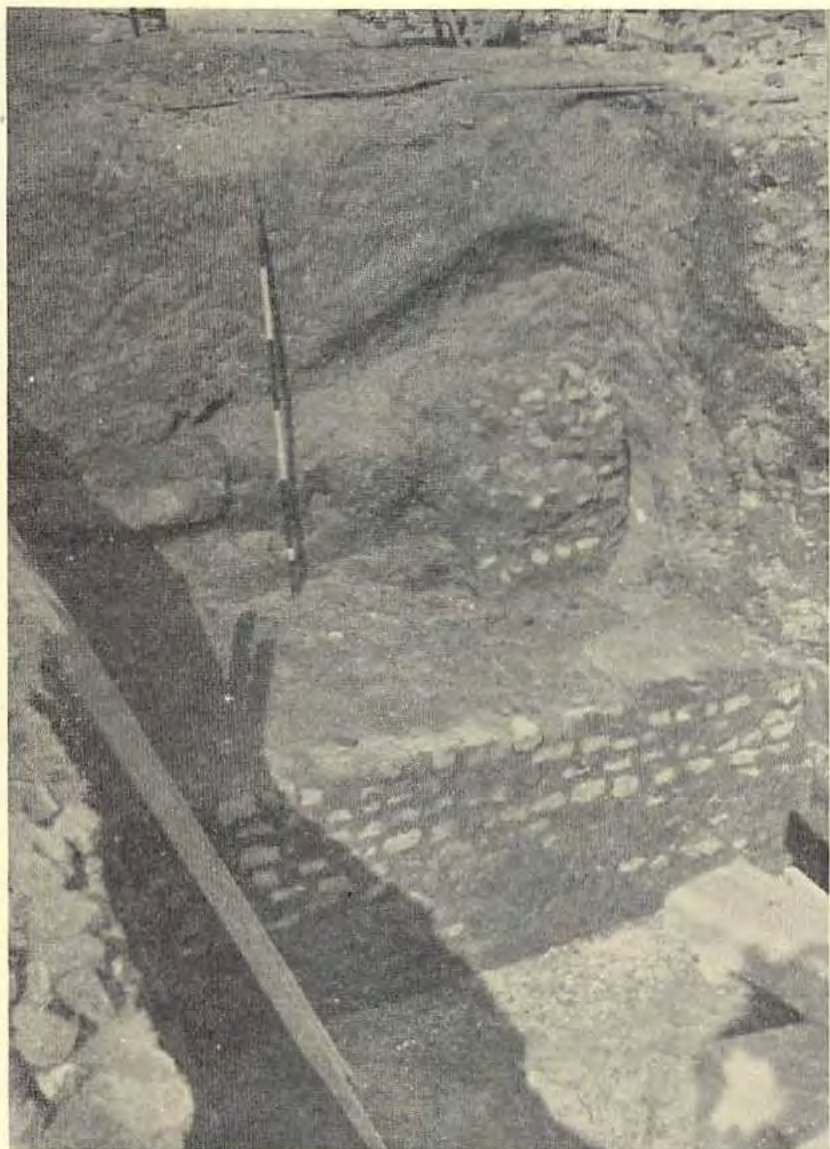
SOUTH FACE OF PLATFORM, WITH PIER 2 AND THE PLASTER MOULDING OF WALL 3 (left).
