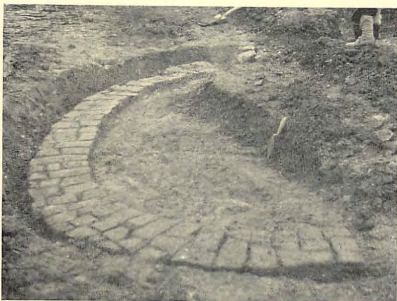
FIG. 3. KILN FOUNDATION, LOOKING NORTH.
