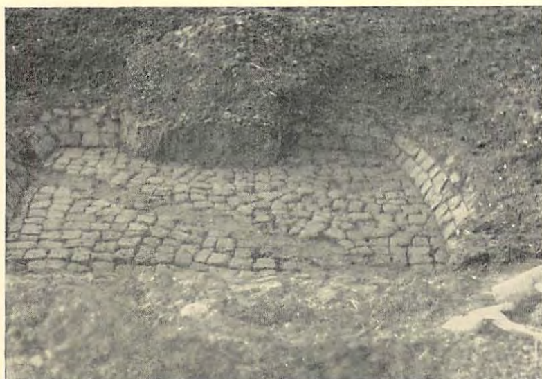
FIG. 17. PUGGING PIT SOUTH OF LATTON STREET, SHOWING SOME PREPARED CLAY IN SITU. DIAGONAL LINE SHOWS SITE OF DRAIN.
