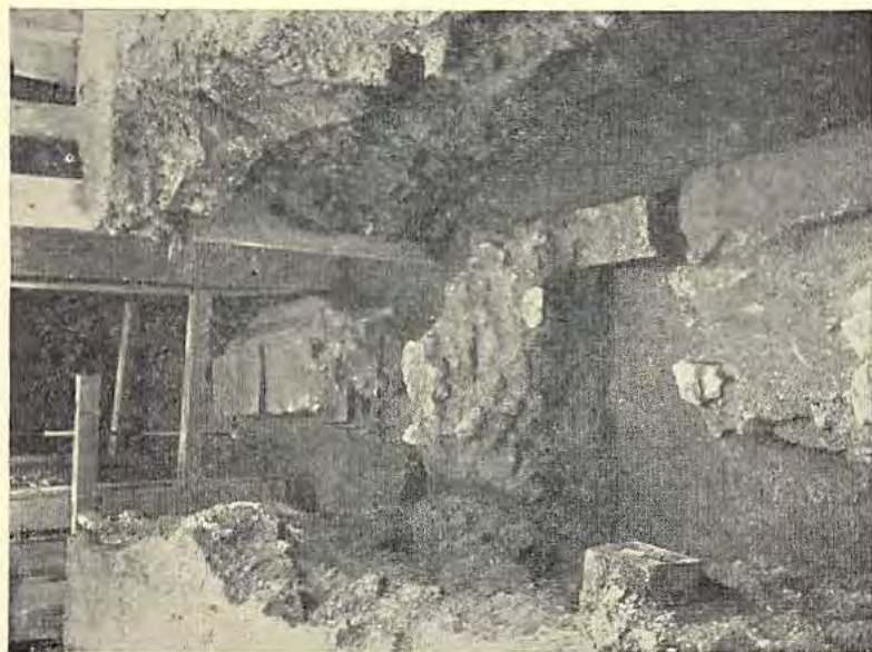
A. PIER 3 AND WALLS, LOOKING EAST.
