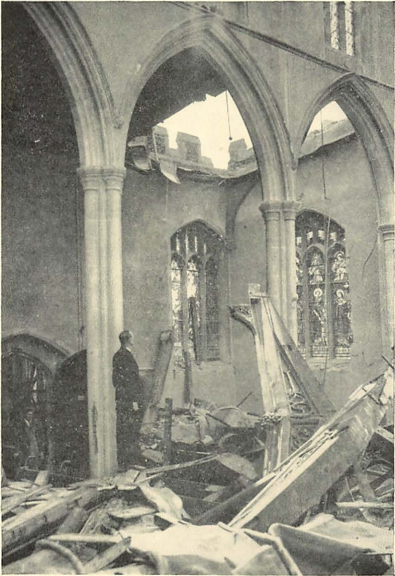
COGGESHALL CHURCH: ROOFLESS WESTERN BAY OF SOUTH AISLE.
