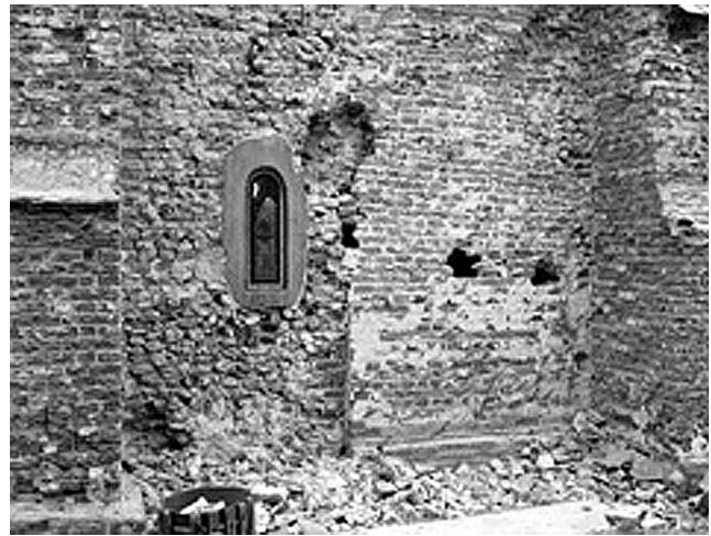
Plate 2 Little Clacton church, the north chancel wall after the removal of cement render.
