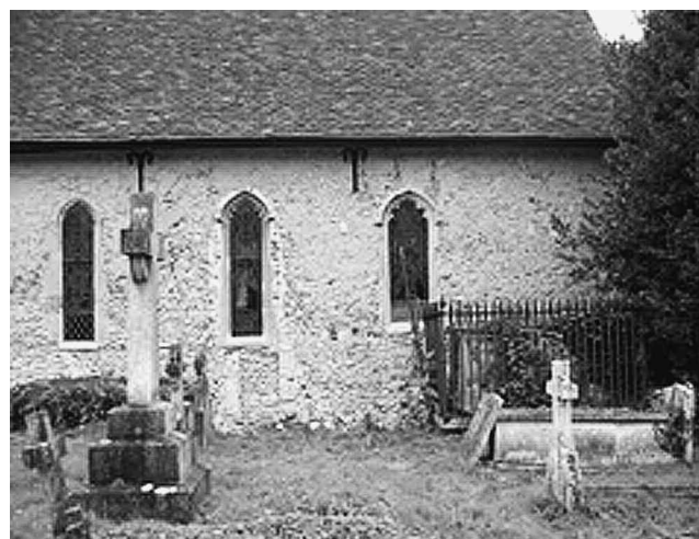
Plate 4 Middleton church, south elevation of the chancel. The Tudor doorway can be seen below the central lancet window which is of Victorian date. The door marks the division between the 12th-century chancel and an eastern extension to it in the 14th century.
