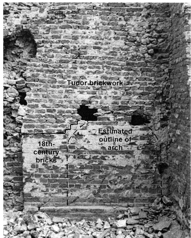
Plate 3 Little Clacton church, an interpretation of the development of the north chancel wall.
