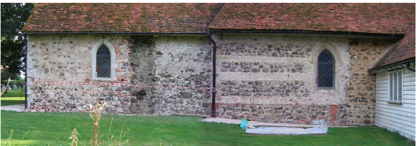
Plate 6 Little Totham church, north elevation with render removed
