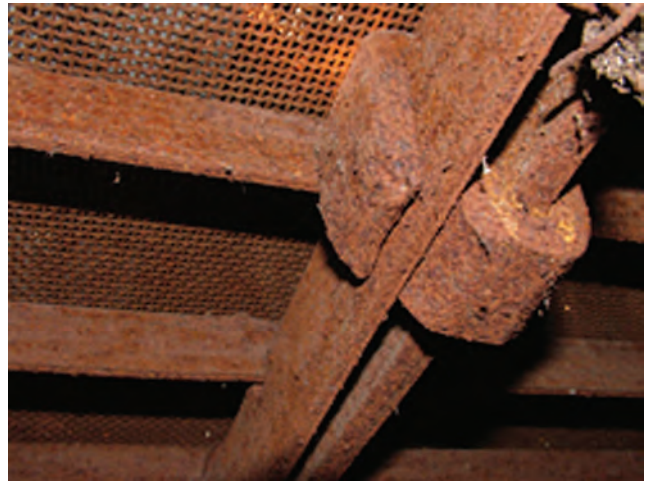
Plate 4 Detail of the construction of the wedge wire floor
