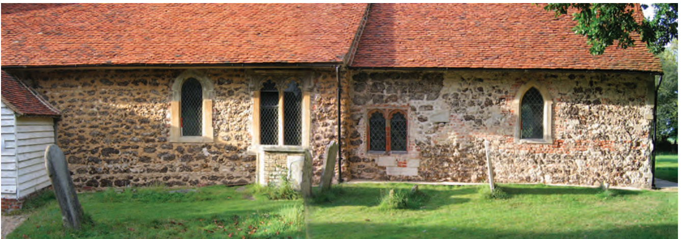
Plate 5 Little Totham church, south elevation with render removed
