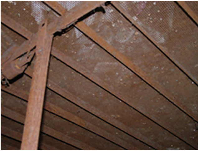
Plate 3 The wedge wire floor in the malting kiln
