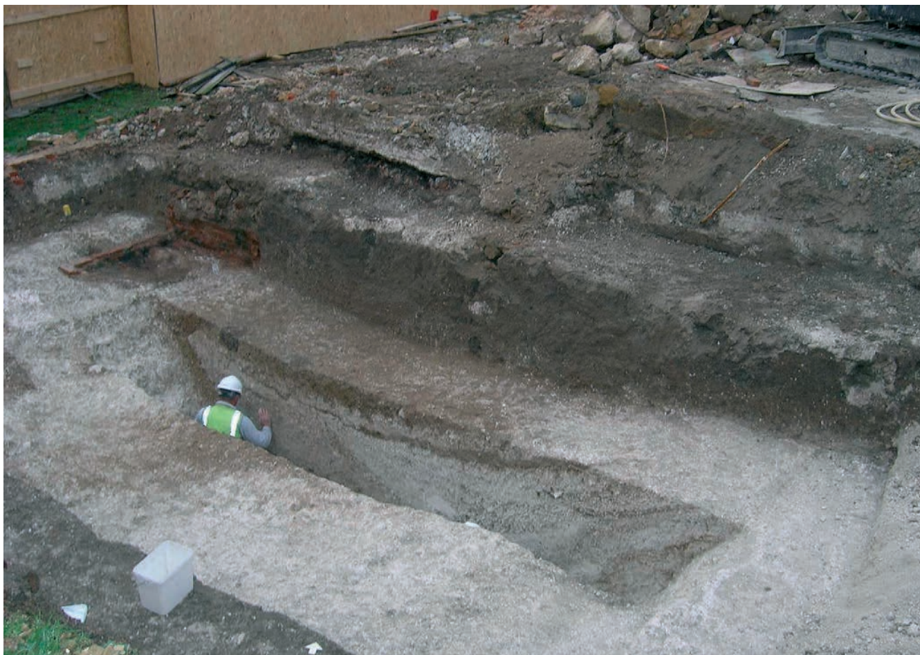
PLATE 1: Excavation of the outer bailey ditch, 63A Castle Street (looking north-east)
