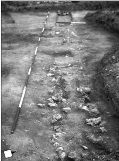
Photo point 1 showing flint foundation of Roman building in Trench F, looking east.
