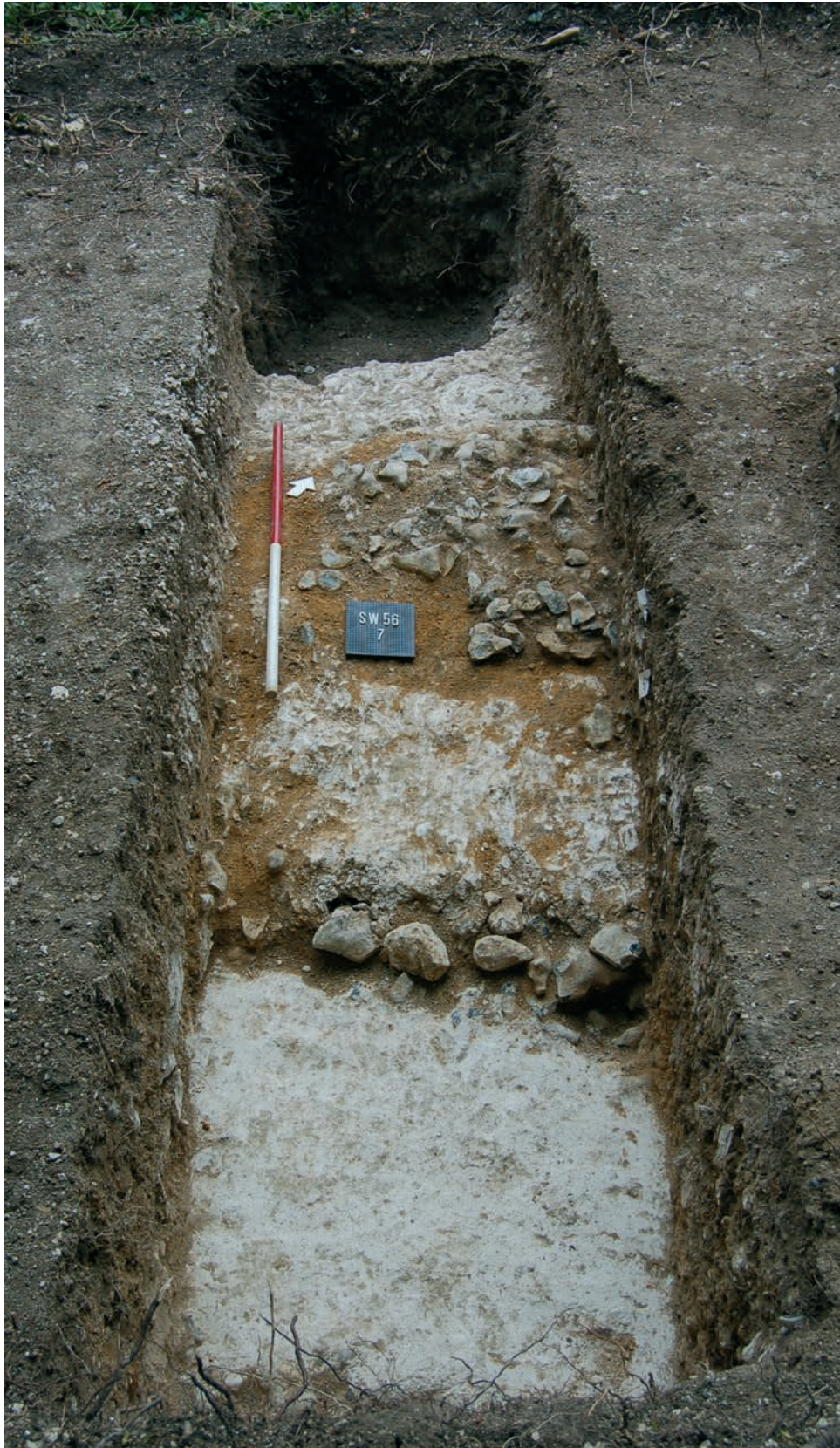
PLATE 2: Wall foundation and bank deposits, r/o 30 Castle Street (looking north-west, 1m scale)
