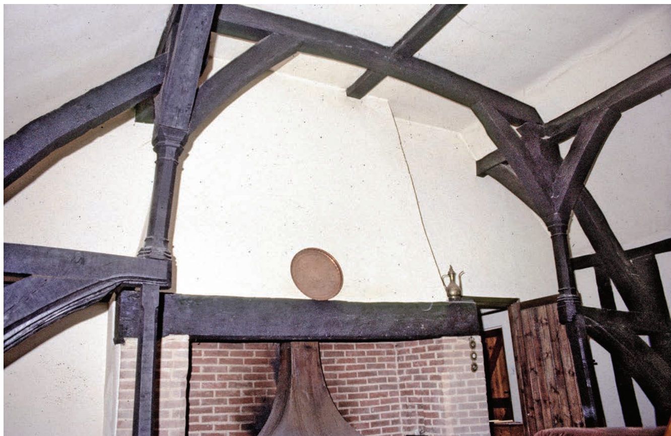
FIGURE 17: North side of centre truss of Gatehouse Farm, Felsted, where the centre of the dropped tie-beam has been cut out and props inserted under the cut ends
