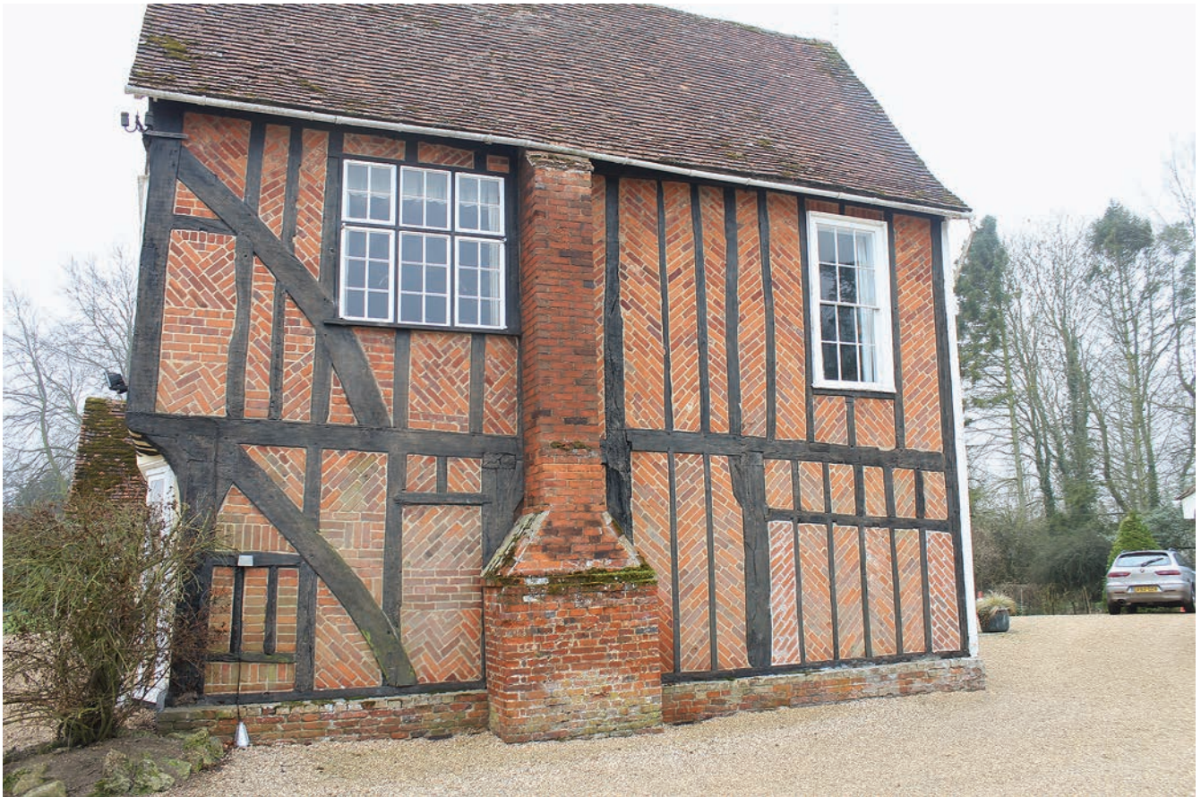
FIGURE 12: East side of high end cross-wing. Jowled posts support ground floor ceiling joists
