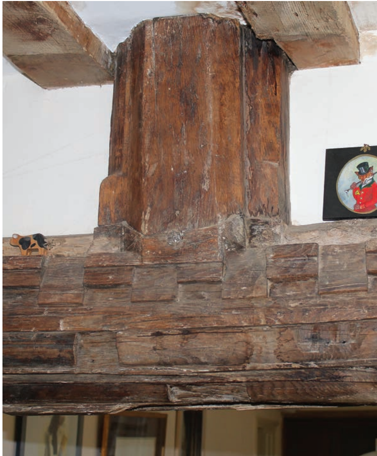
FIGURE 9: Base of north raised arcade post
