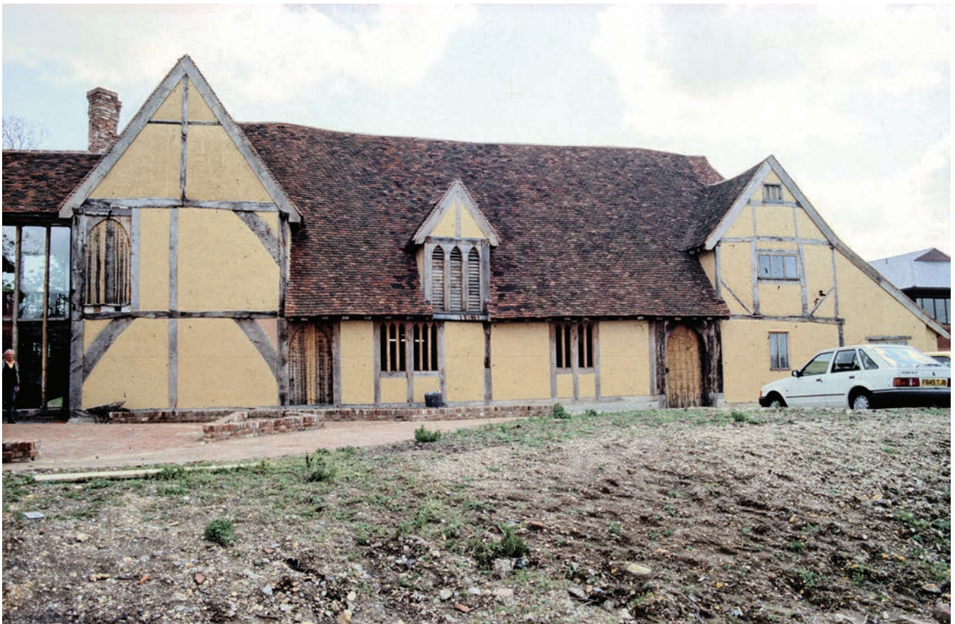
FIGURE 13: Rear of Upton Court, Slough, Berkshire, an aisled hall dated to 1320d (V&A 19, p. 46), showing external 1st floor door to parlour chamber
