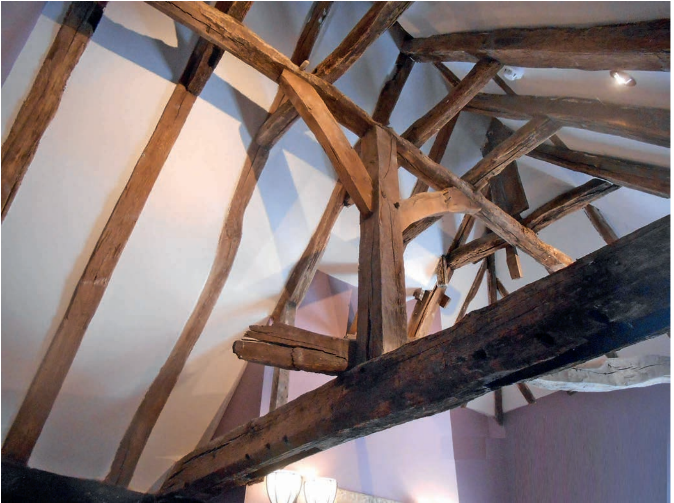
PLATE 2: Crown-post roof in the eastern cross-wing. Photograph by Tim Howson, 2015
