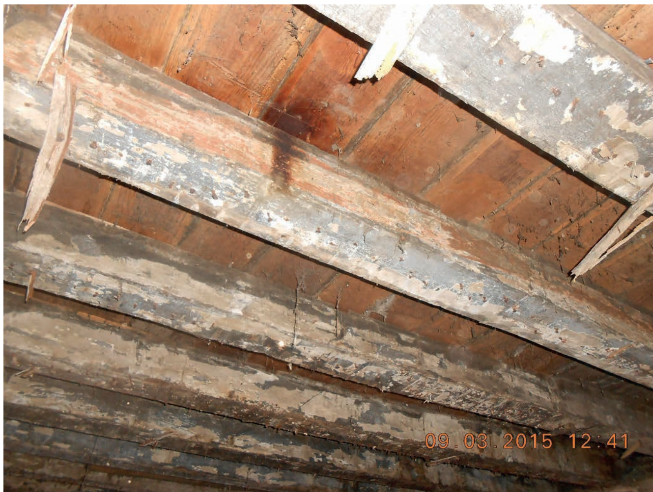
PLATE 3: Seventeenth-century grey paint on floor joists in the western hall range. Photograph by Tim Howson, 2015.
