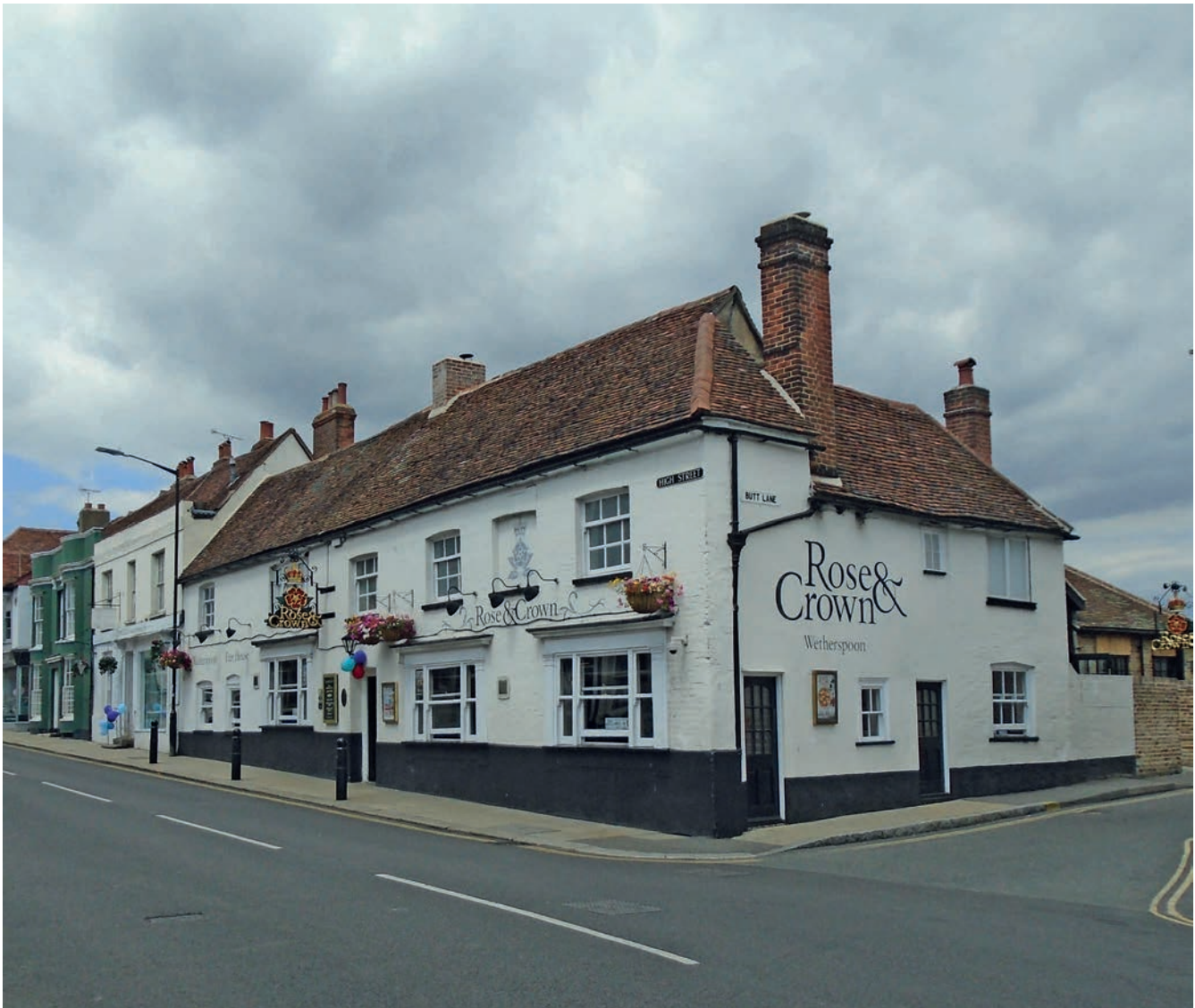
PLATE 1: High Street and Butt Lane elevations of the Rose and Crown. Photograph by J. R. Smith, 3 July 2019
