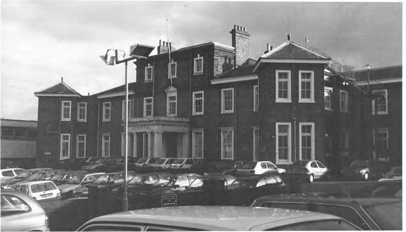
Plate 5 A view of the original 1819-20 Late Georgian hospital building at Essex and Colchester General Infirmary showing two of the later Victorian (1879-80) diagonally set sanitary blocks.
