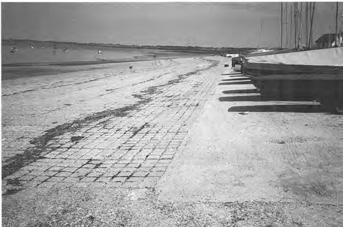
Plate 11 The concrete hard at The Stone, on the River Blackwater, built to accommodate four Landing Craft, Troops, in preparation for the D-day Normandy landings.
