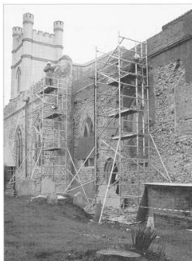
Plate 1 Rivenhall, St. Mary and All Saints, the south elevation as exposed after the removal of cement render (photo A. Letch).
