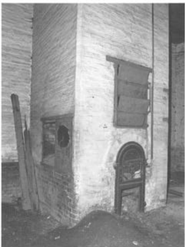
Plate 8 Malthouse No. 3, kiln furnace.
