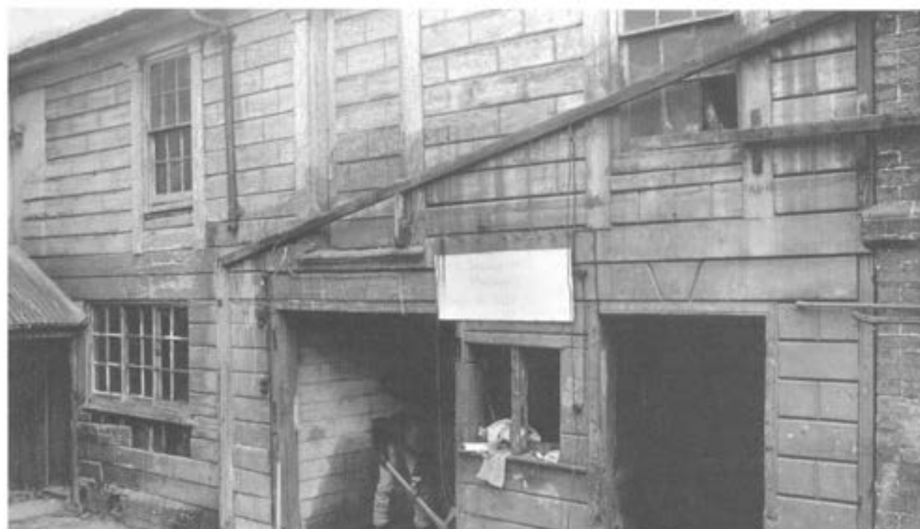
Plate 3 The outbuilding with rusticated weatherboarding to the rear of the listed shop on Market Row, with work in progress on trench 1.
