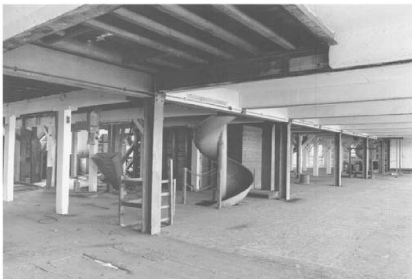
Plate 4 Malthouse No. 2, second floor, showing sack chute, other hatches, and screening machinery.
