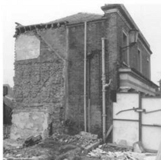
Plate 2 The listed shop on Market Row after the demolition of the back half of the double-pile building and the swimming pool and toilets, showing the impression of the end truss of the 16th century timber building in its side (looking west).
