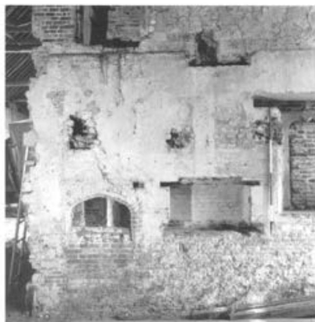
Plate 3 Rochford Hall Barns, interior of the west wing, looking north (1985). Note first-floor fireplace, sockets for common joists, doors into north-west corner tower, and scar for wall dividing west and north wings.
