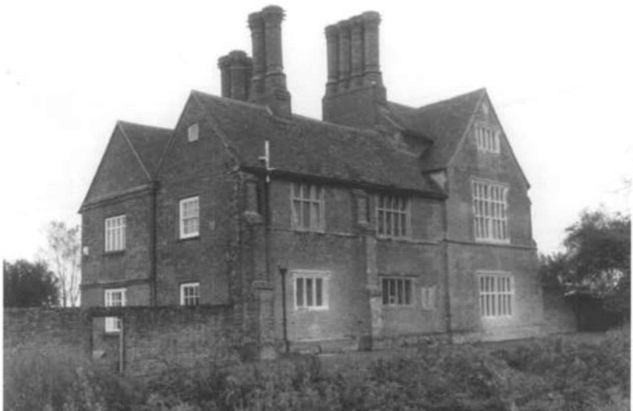
Plate 1 Wimbish, Broadoaks, the north and east elevations.
