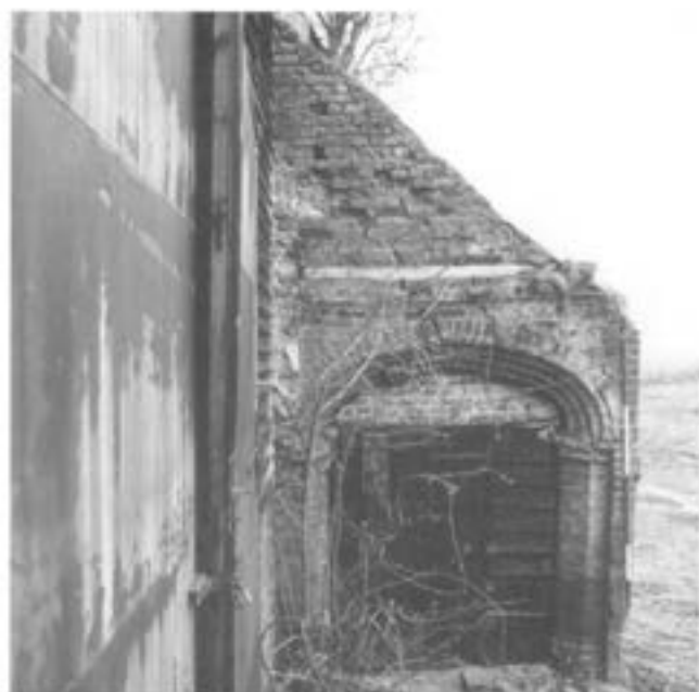
Plate 5 Rochford Hall Barns, arch in the south wall of the wing that formerly adjoined the central wing (1985).
