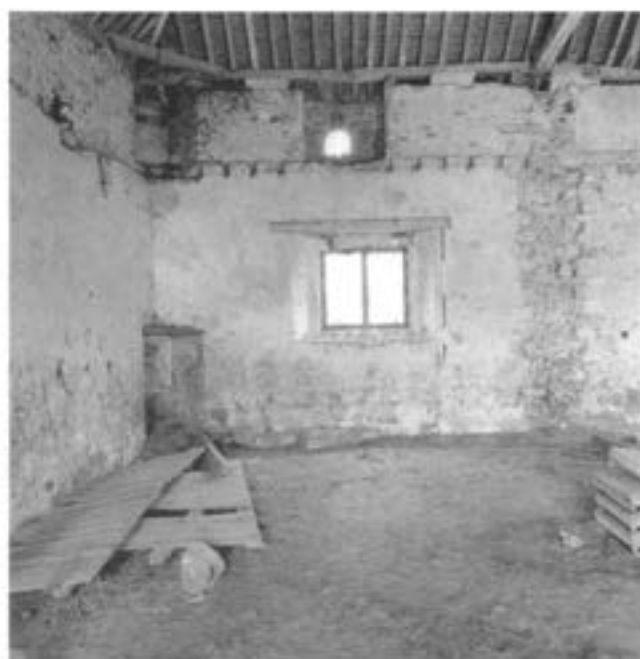
Plate 4 Rochford Hall Barns, interior of the west wing, north end of the east wall, showing original plaster, joist hole for first floor, niche, and blocked door to stair turret (1985).
