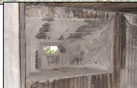
Plate 2. The FW3/28a 2 pounder anti-tank pillbox to the south of Broomfield Mill (SMR 10872). Inset, a detail of a 'crenellations' and an interior view of a loop-hole for a Bren LMG.
