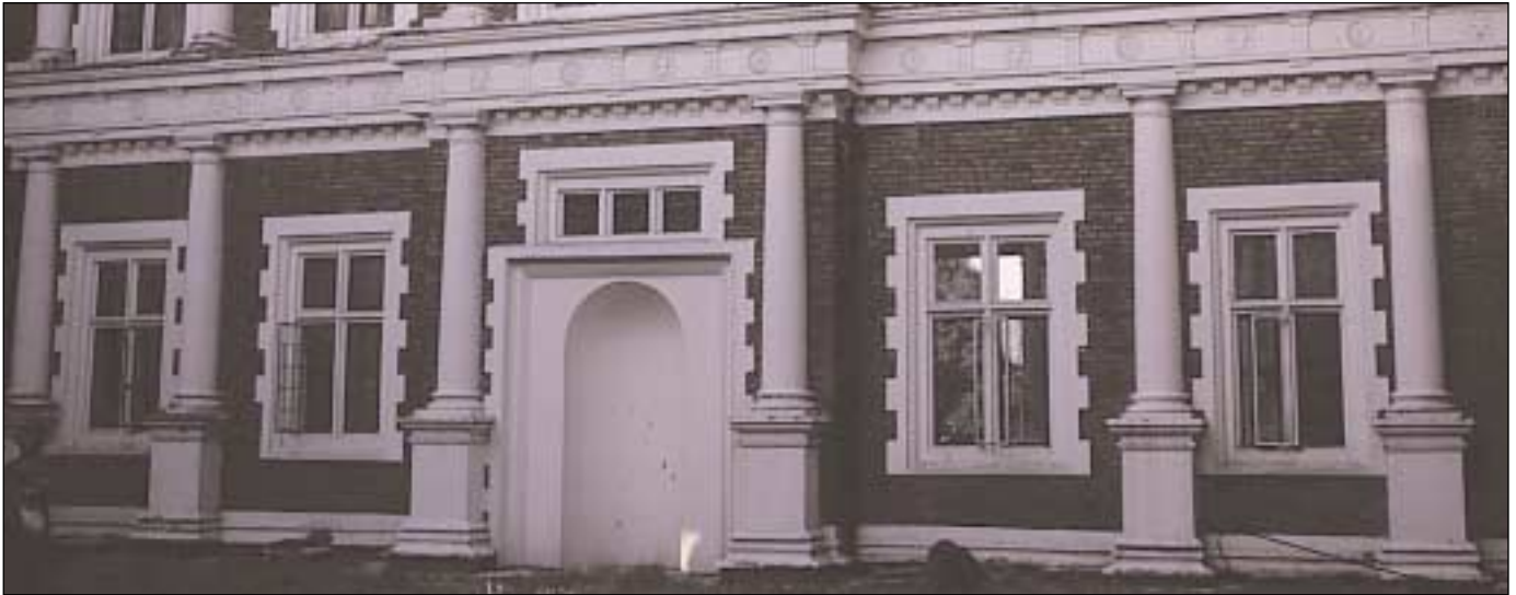
Hill Hall, Theydon Mount. East Block of Inner Courtyard. (Courtesy of John Boyes).
