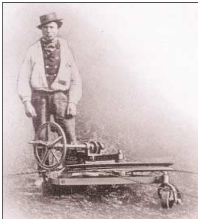
Light travelling anchor of steam plough.
