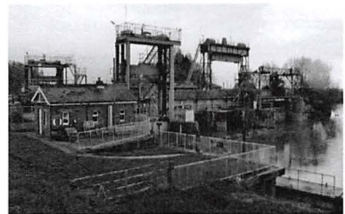
AG Wright sluice, 2012
