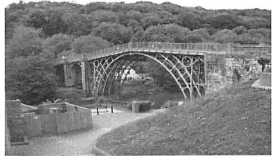
Cast iron bridge at Ironbridge. Photo supplied by Peter Wynn.
