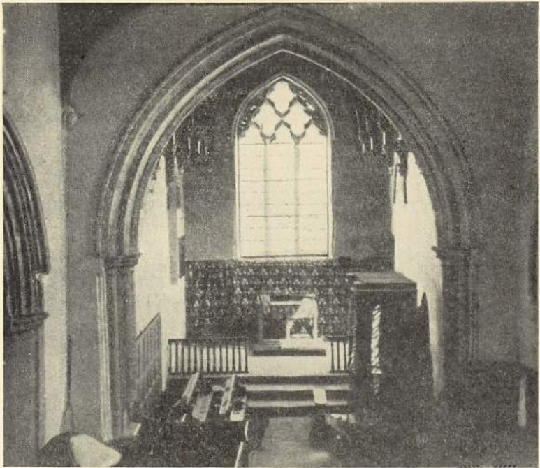
Fig. 1.—Chancel, looking east. (Before Rebuilding.)
