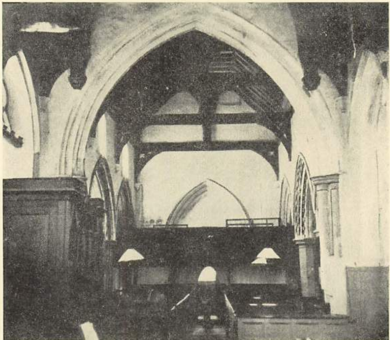
Fig. 2.—Nave, looking west. (Before Restoration.)
