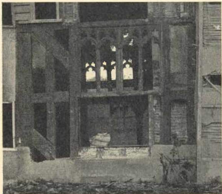
Fig. 1.—MANOR FARM (formerly Cabborns), STANFORD-LE-HOPE: OAK WINDOW-FRAME, DISCOVERED IN SOUTH-EAST WALL OF HALL IN 1940, XV th CENTURY.
