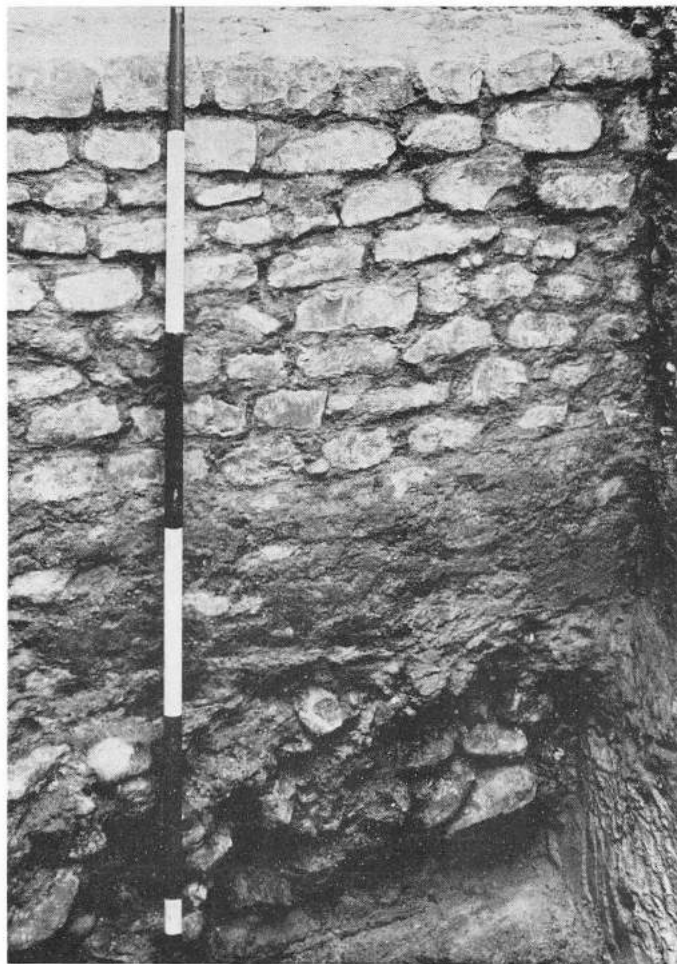
Plate IIIa Foundation Platform of South Arcade
