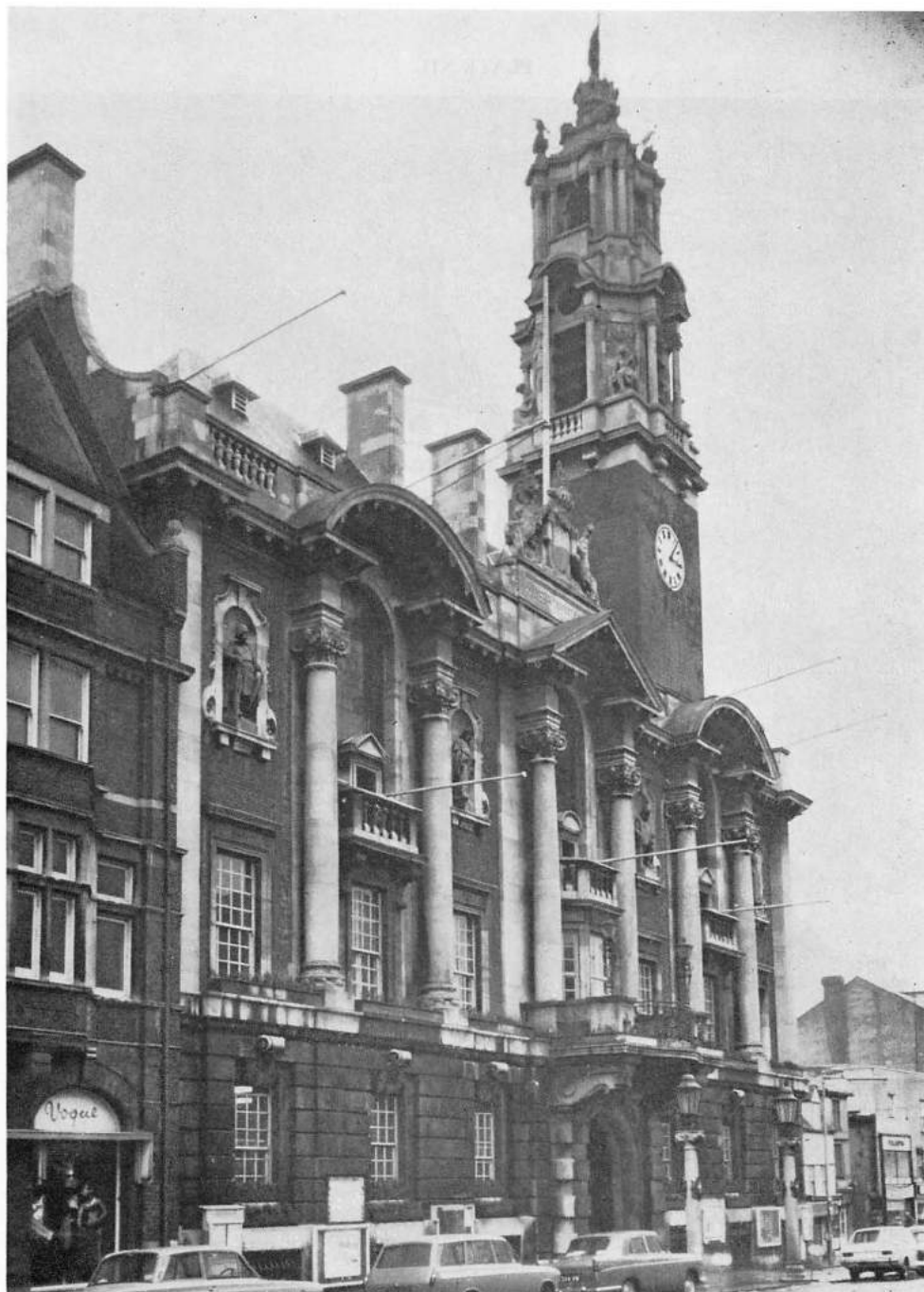
John Belcher, Colchester Town Hall (designed 1897, built 1898-1902).
