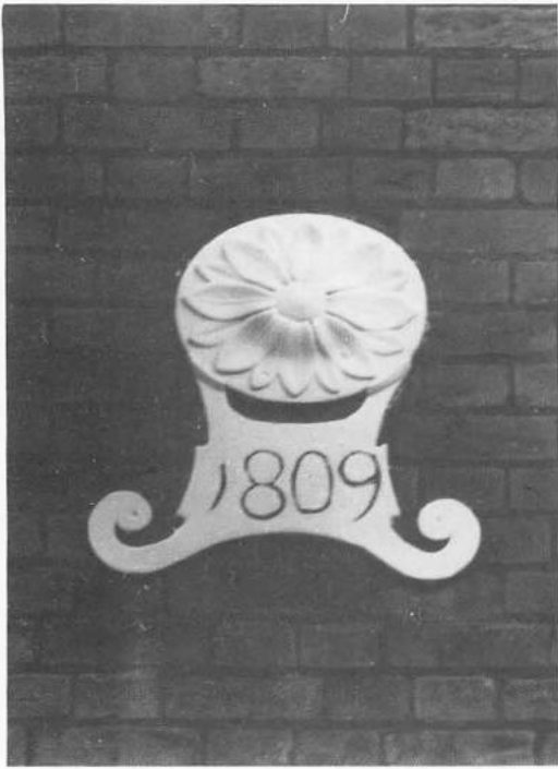
This dated foliated tie-plate on Wallis's house at 5 North Hill, Colchester, serves no functional purpose, and was doubtless both ornament and advertisement. Presumably the oldest surviving casting from an Essex foundry, some 18 tie-plates from the same pattern can be found in Colchester, Wivenhoe, Rowhedge, Dedham and East Bergholt.
