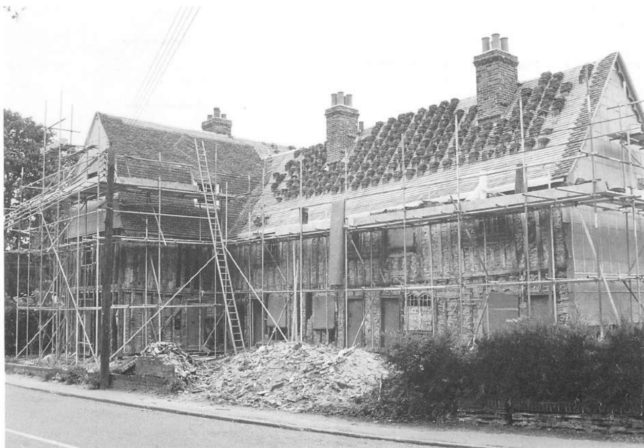
Plate 1 The timber frame exposed during reconstruction.
