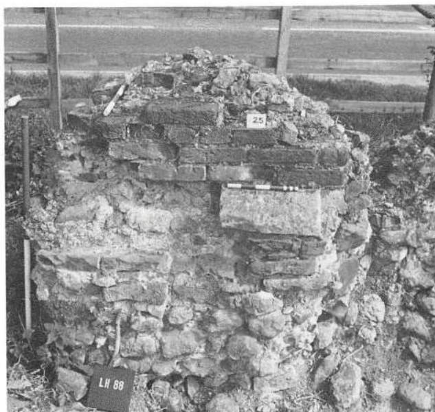
Plate 3 The buttress at the north-east corner, showing later repairs. Horizontal scale in centimetres and decimetres.
