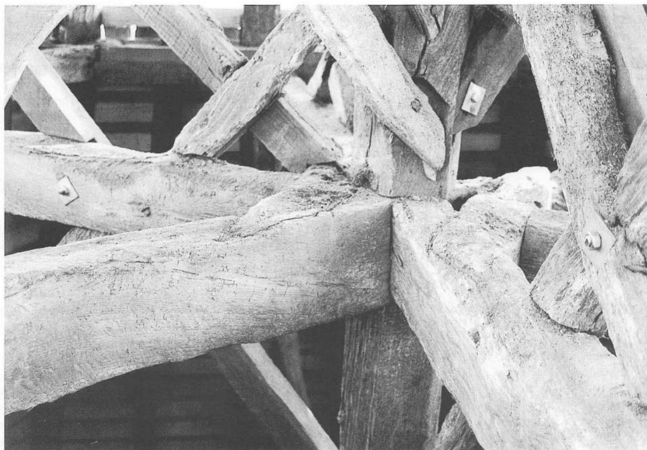
Plate 5 Wheel centre at first lift showing crossing spokes, housed tying pieces with spokes mortised in. Spire braces passing through wheel with halved and pegged joints. Base of spire mast for second lift controlled by these braces from below.
