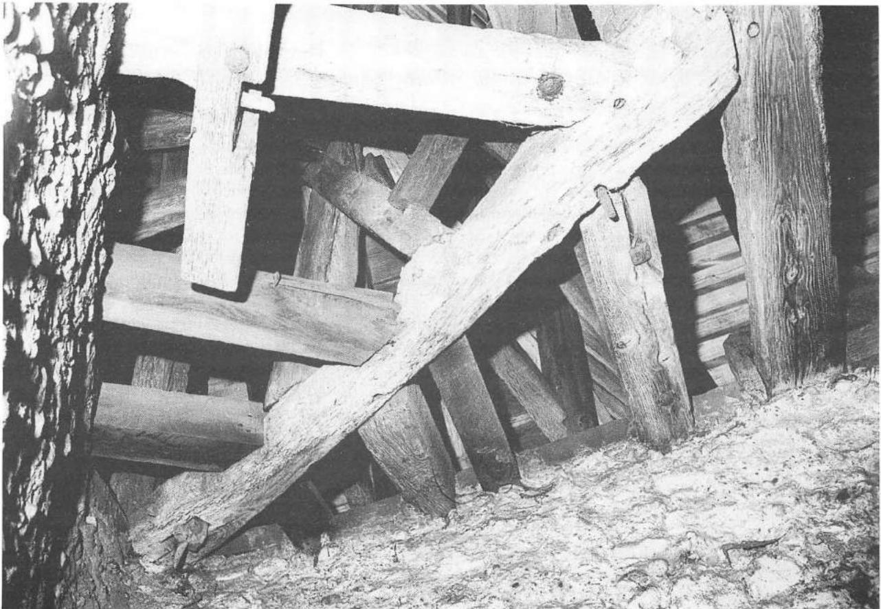
Plate 3 Underview of spire floor to north corner. Sub-spine to north spirelet, rafter beams and cut-off top beam of underframe pegged to floor. Empty notched lap joints in top beam and sub-spine.
