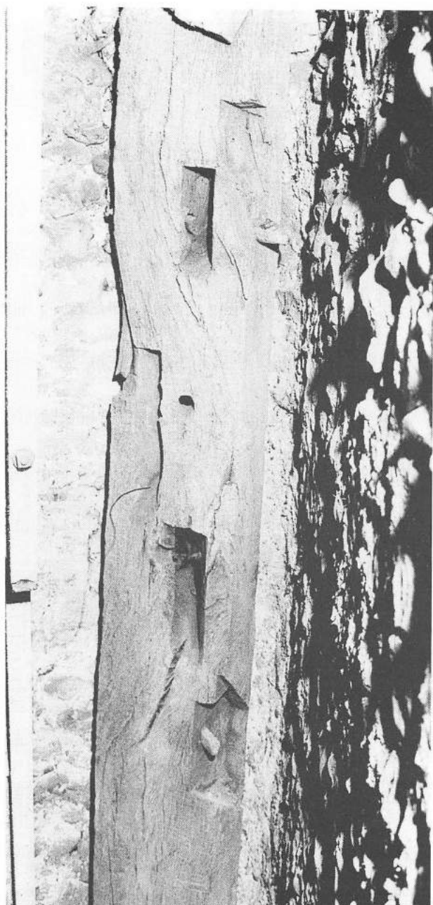
Plate 1 Spire underframe. West corner post showing from top. Square-cut mortise, angle mortise to left, angle mortise to right and notched lap joint.
