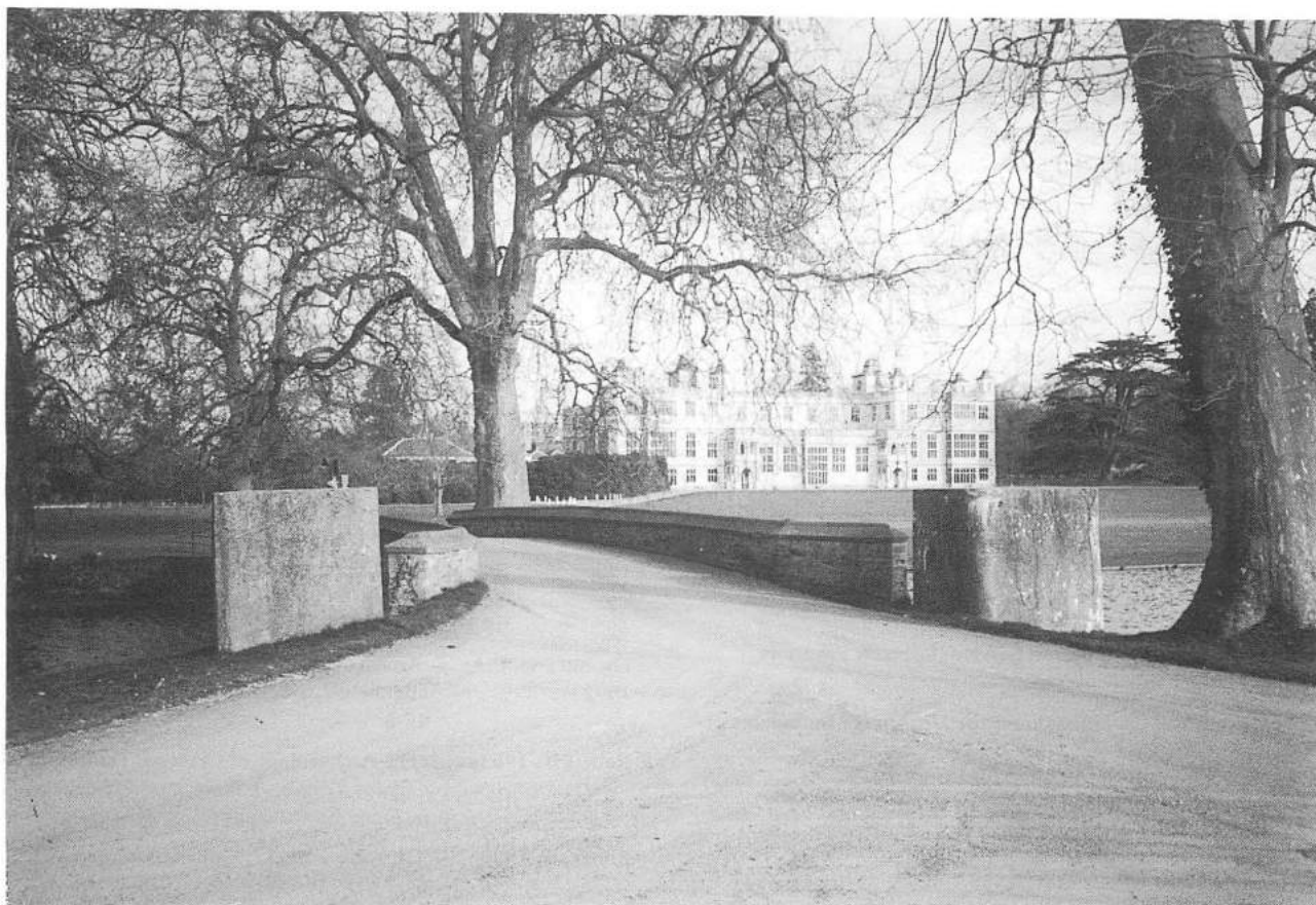
Plate I Anti-tank blocks astride the Stable Bridge at Audley End (a heavy steel cable was originally stretched between them and anchored at each end).
