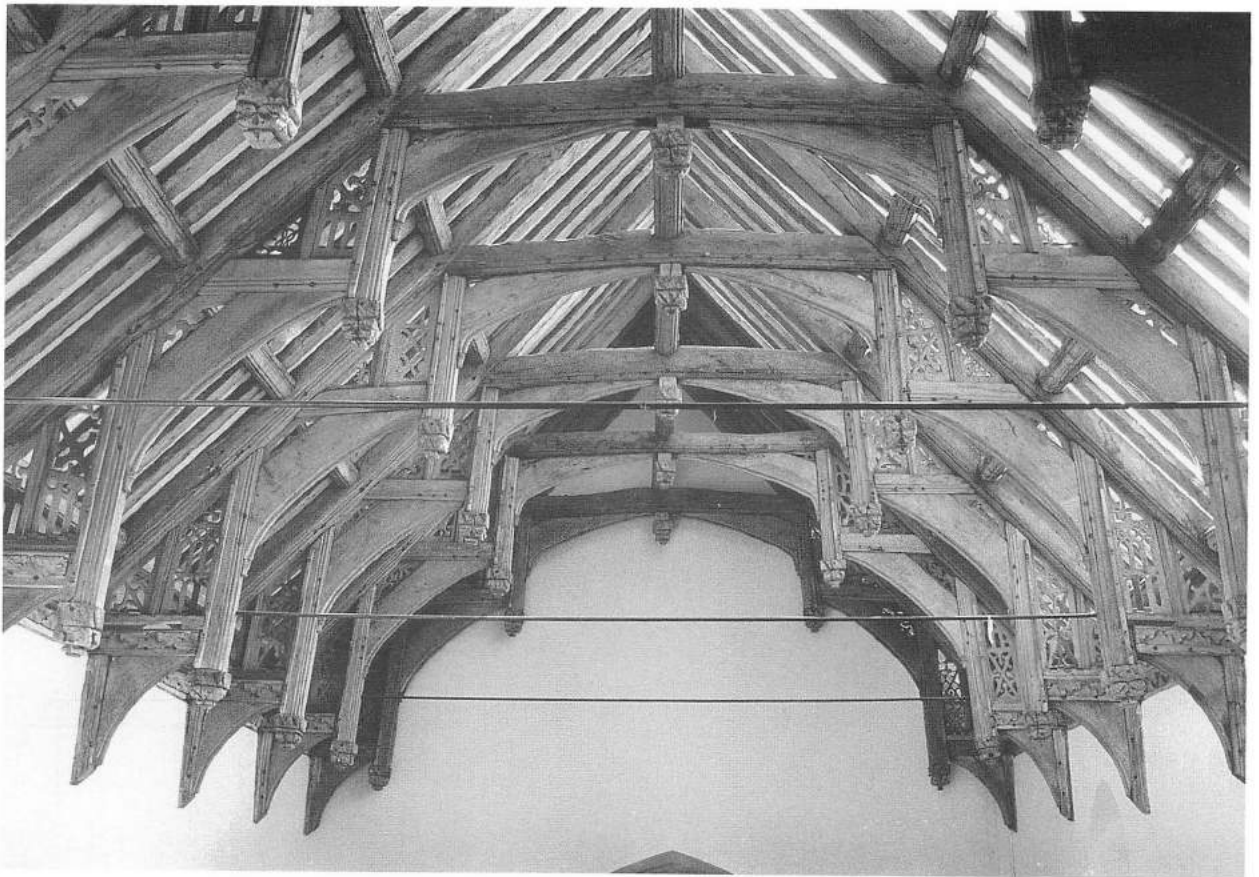
Plate 3 Gestingthorpe St Mary; the hammer-beam roof of c. 1500. The church was retiled in 1995.
