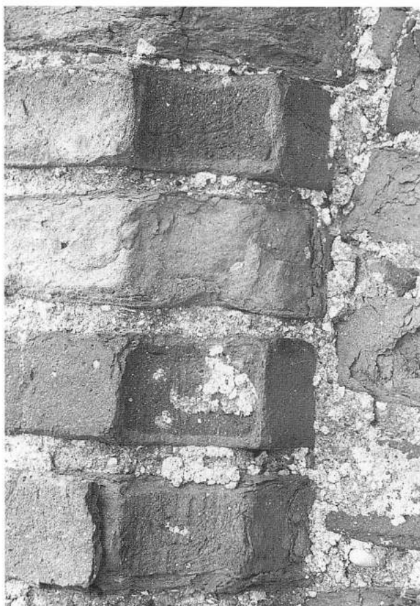
Plate 2 South window jamb clearly showing the rubbed replacement bricks, two of which have a black core as with original Coggeshall bricks
