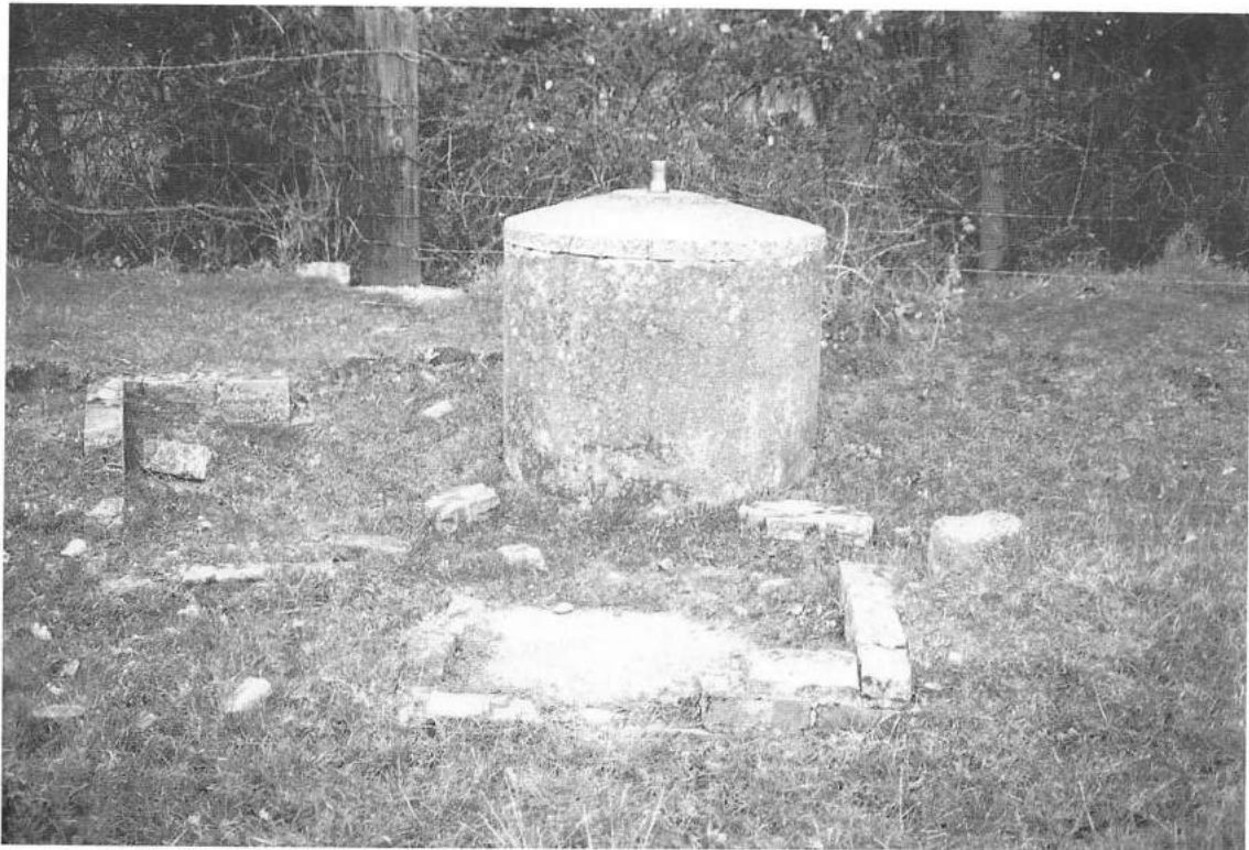
Plate 2: Spigot Mortar Pedestal at Tilty with the remains of its ammunition alcoves (Photo by Fred Nash).
