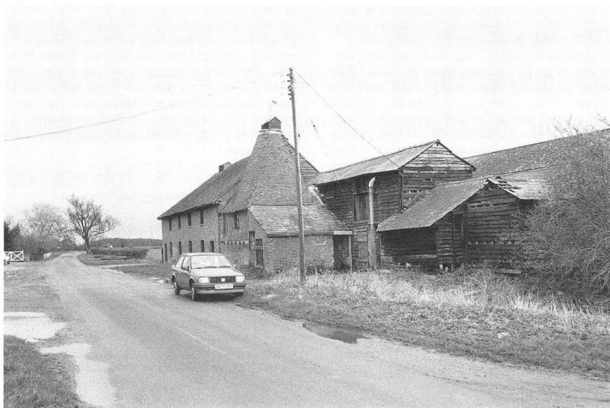
Plate 3 Gowers Farm Malthouse, Stisted. Barley was delivered at the far end of the building and progressed toward the kiln; the finished malt was then stored in the weather-boarded range on the right.
