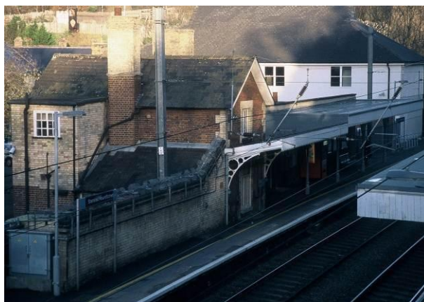
Down side platform showing 1845 station building and the two canopies of different designs, reflecting the different dates of construction.
