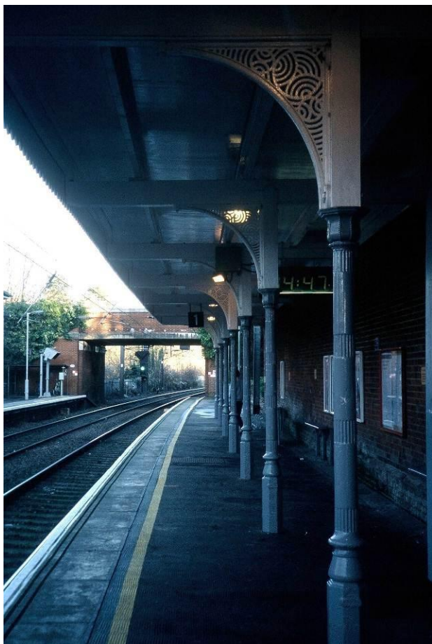
Up side platform showing detail of the 1889/90 columns and brackets supporting the canopy. The columns are round in section on an octagonal base with four short lengths of fluting on the main portion of the column.
