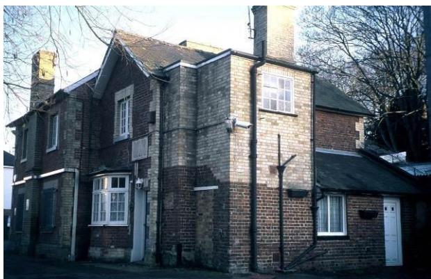
Stansted Mountfitchet station building of 1845, the original building being the gable end on the right.
