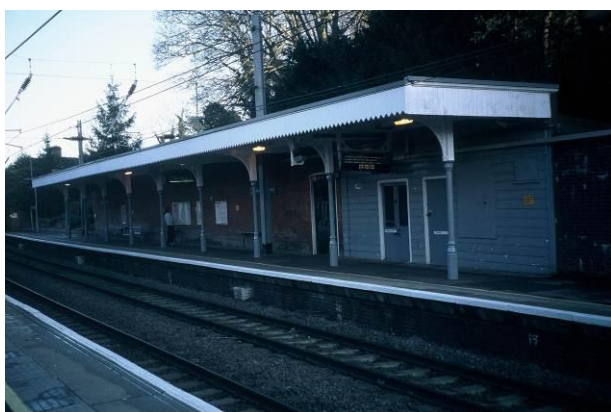
Up side platform with timber clad waiting room and canopy of 1889/90 supported on cast-iron columns.
