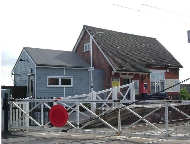
Up-side brick booking office and timber level crossing keeper's hut on the up platform.
