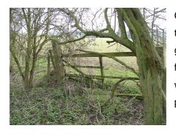
Crossing point comprising four concrete gate posts, two either side of the cutting and a pair of timber gates. The crossing is banked slightly along its flanks suggesting its was used as a cattle drove way. The gates have deteriorated but the concrete posts remain upright and intact.
