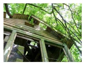
5827 4499). The signal box is a two-storey, rectangular plan building with gable ends east and west and an external straight flight to the first floor. The walls are clad with weatherboard (shiplap) nailed onto a heavy primary braced 3 bay softwood (pine) timber-frame mounted onto a 5 brick course 1B wall plinth capped with chamfered blue brick copings. Heavy iron brackets with quatrefoil
