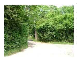
The embankment, brick revetment and piers belonging to the bridge remain either side of the Hadstock Road, but the deck of the underbridge (probably iron beam) has been removed. The remains are currently overgrown but show little obvious signs of distress.
