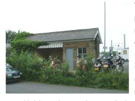
The original branch line halt and a length of platform still survive to the south-east of the main station building and at the western extreme of the former branch line. The waiting room/station office (EHER 40454) is a small unimposing building lacking the grandeur of the main station. It is built using a similar yellow stock brick in Flemish bond and uses blue bull-
