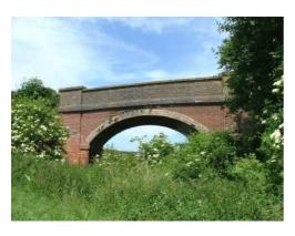
Bond, a three course on-edge brick arch with white brick dressings and red brick piers and splay revetments holding back banks to the north and south. The brick parapet, tops of the piers and saddle-back copings are later replacements. The bridge remains in use, now providing access to farm buildings to the west of the line and is well maintained, showing areas of recent repair, particularly to the revetment walls.
