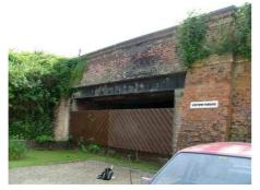
Iron beam and brick jack arched bridge supported on piers of red stock brick with yellow brick dressings and a parapet with decorative bands and over-sailing brick copings. Four jack arches support the bridge bed axially and spring from five large wrought iron bridging beams, manufactured in 1864 by founders J.I. Headley of Cambridge. The outer
