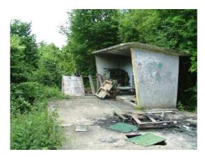
Built in 1957 for the benefit of the Acrow Works and particularly its staff, Acrow Halt still lies within a stretch of overgrown cutting to the east of the works and north of Ashdon Road. The Halt comprises a c. 80m stretch of reinforced concrete platform ramped at both ends and oversailing the former line to the east. A simple lean-to shelter of concrete construction is situated along the
