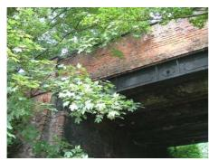
specifications as its contemporary to the west at Debden Road. It is an Iron beam and axial jack arched bridge supported on brick-built piers of red stocks in English bond, with yellow brick dressings and a brick parapet. Four jack arches strengthen the deck axially and spring from five large original wrought iron I section bridging beams. The outer
