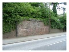
Former iron beam underbridge spanning Thaxted Road. The bridge deck was probably removed due to the height restrictions it imposed upon one of the main arteries serving the industrial area of the town. All that remains is the red brick piers, earth embankment and the brick abutments. The brickwork is much plainer than that used in the
