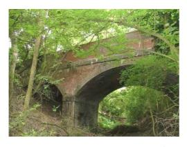
A triple arch accommodation bridge built with a large central (rail) arch flanked by smaller outer arches springing from the railway banks. Built with red brick piers and abutments (English bond), the bridge has white brick dressings facing each of the three course on-edge arches and a plain blue brick band at deck level. The parapets, also in red brick, are modern and
