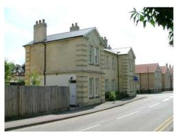
Built in c.1865 the station is a symmetrical 2 storey 5 bay building in yellow gault brick, with forward set gabled cross-wings at each end. The shallow pitched roofs are slate covered and the angles are dressed with nail-head banded brick quoining (a characteristic of the SWRC) rising to a simple moulded eaves cornice and an open pediment at gable. The walls have a
