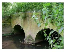
A brick-built C19 culvert channelling the River Cam below the railway embankment to the north-east of Wendens Mill. The bridge abutments and revetments are built in red stock brick laid in English Bond while the parapets are capped with blue brick copings. The doublearch of the culvert is built using four on-edge courses, and is supported on a central
