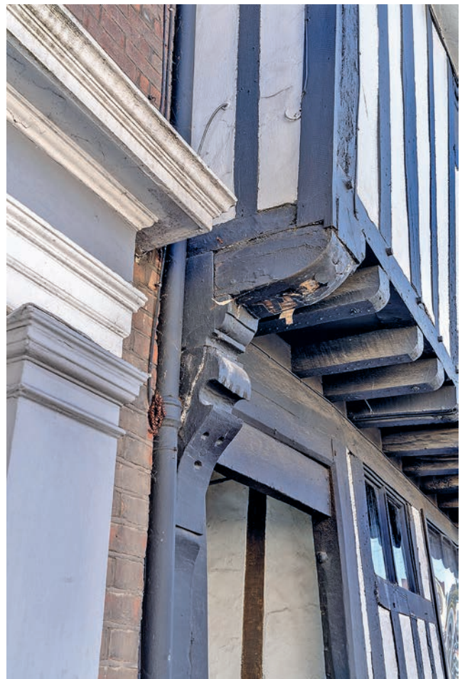
FIGURE 45: Decorative jetty bracket on the east side of 17 East Hill (corpus no. 8), which probably relates to an adjoining building
