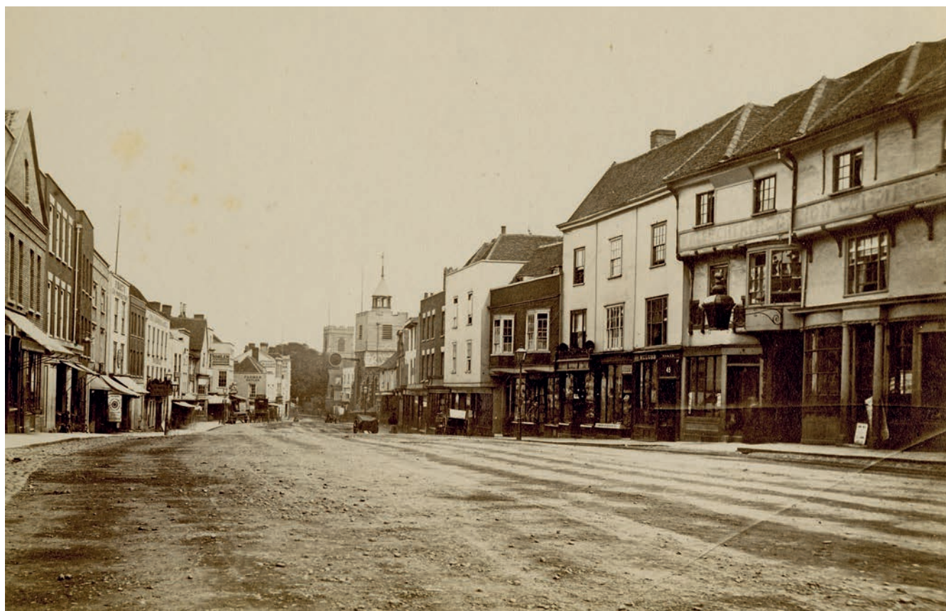
FIGURE 150: View looking east along High Street, early 1870s. The Red Lion Hotel (corpus no. 32) is in the right foreground. The photograph was taken before St Nicholas' Church (centre) was rebuilt with a spire in 1875. Courtesy of Colchester and Ipswich Museums
