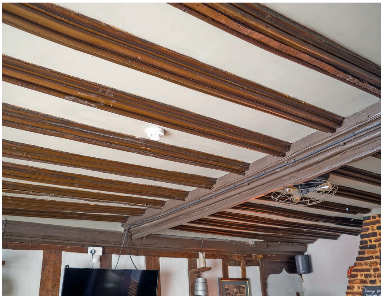
FIGURE 71: Inserted 16th-century moulded floor in The Goat and Boot, 70 East Hill (corpus no. 15). There is a small ogee-headed door at the north end of the west wall, which relates to an earlier cross-wing (to the west). Jess Tipper
