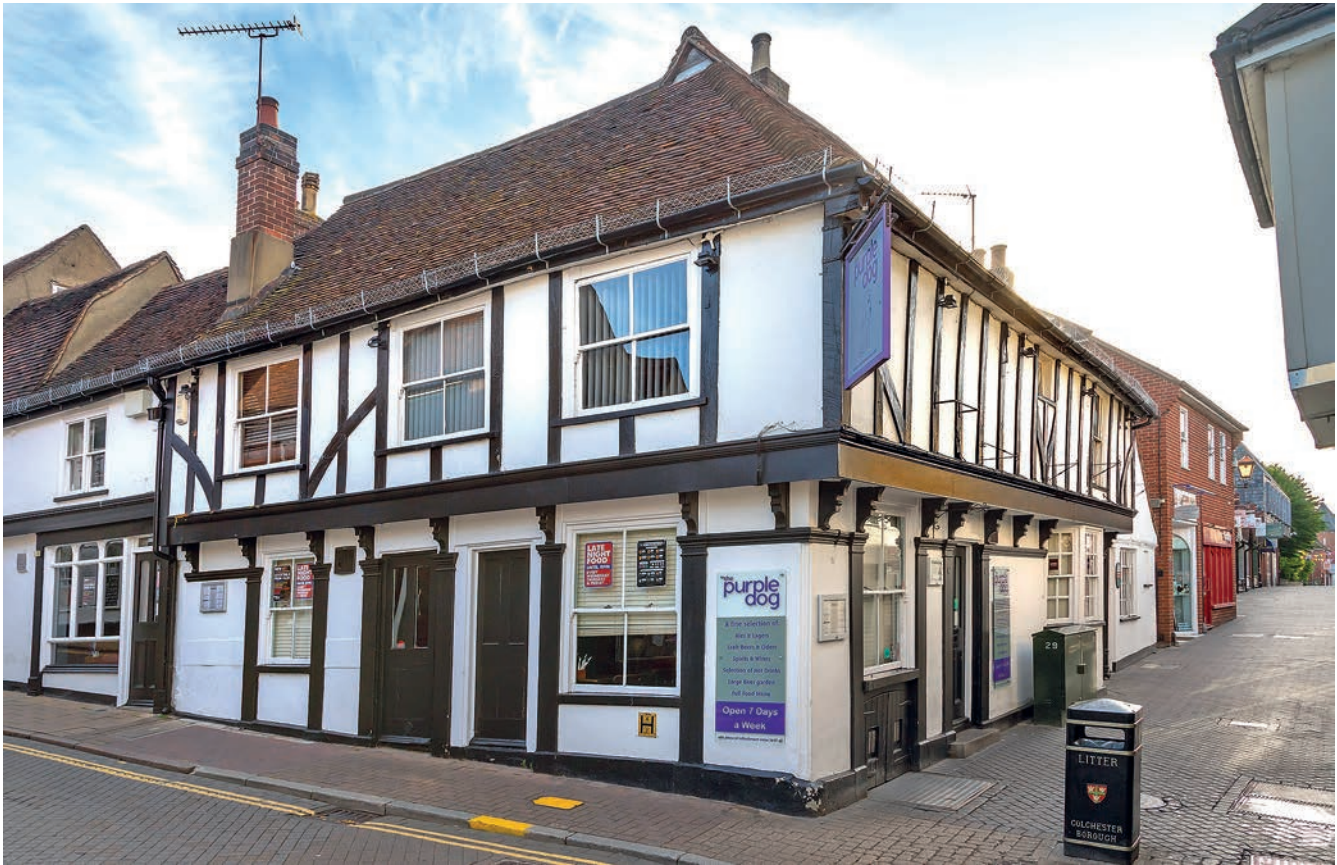
FIGURE 124: 42 Eld Lane (corpus no. 27). The Trinity Street frontage was originally gabled
