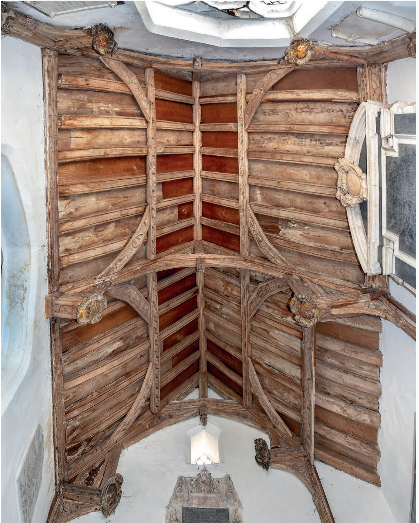
FIGURE 25: Interior of the Audley Chapel, St Michael's Church, Berechurch Hall Road, showing the fine hammerbeam roof (corpus no. 2)
