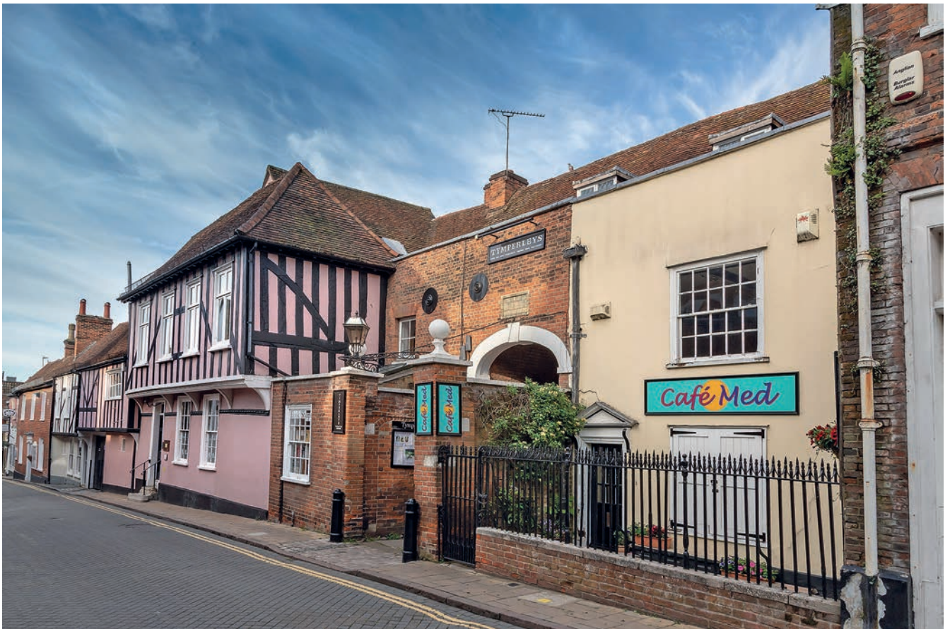
FIGURE 351: 7–9 Trinity Street, Tymperleys (corpus no. 93). The later brick carriage arch is in the centre
