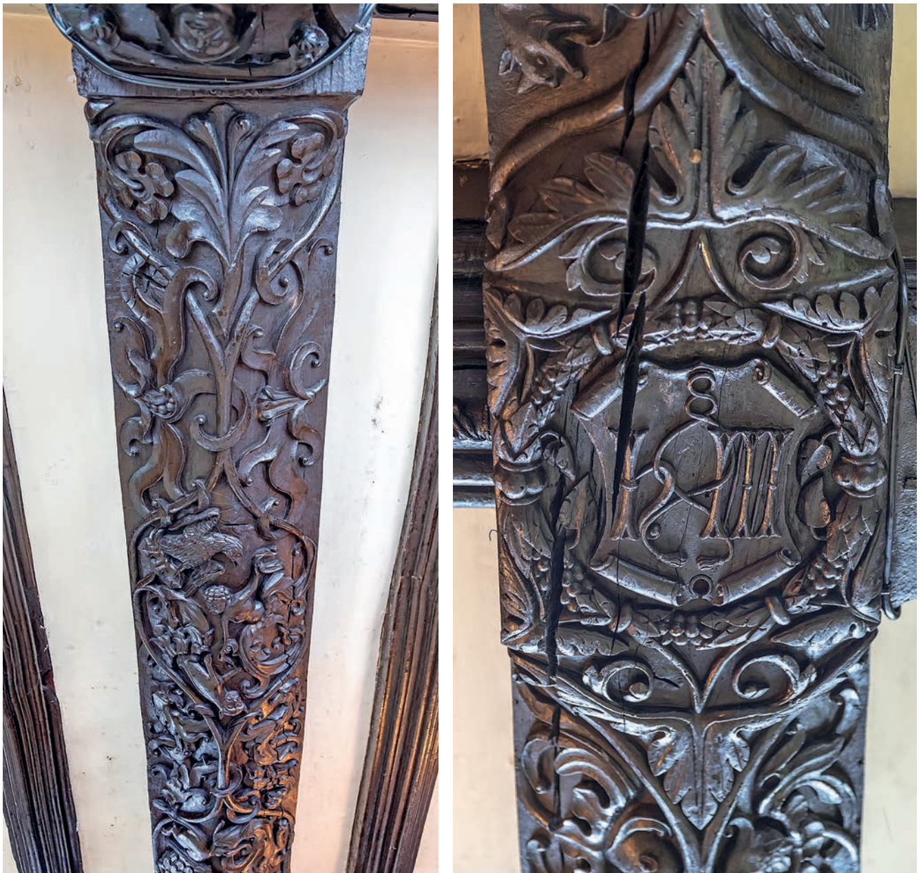
FIGURE 258: Intricately carved bridging joist (and moulded joists), (left) a. in the rear wing of The Marquis of Granby, 24 North Hill (corpus no. 66), (right) b. detail of the bridging joist. The central boss has a shield that appears to bear the initials H.M. or W. intertwined with a knot
