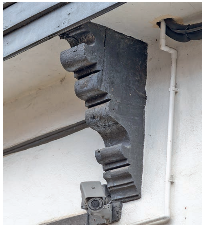
FIGURE 277: Horned jetty and gable brackets, (left) on 46 North Hill (corpus no. 69) and (above) detailed image of a jetty bracket. Notice also the frieze windows on the first floor, suggesting an oriel window in between
