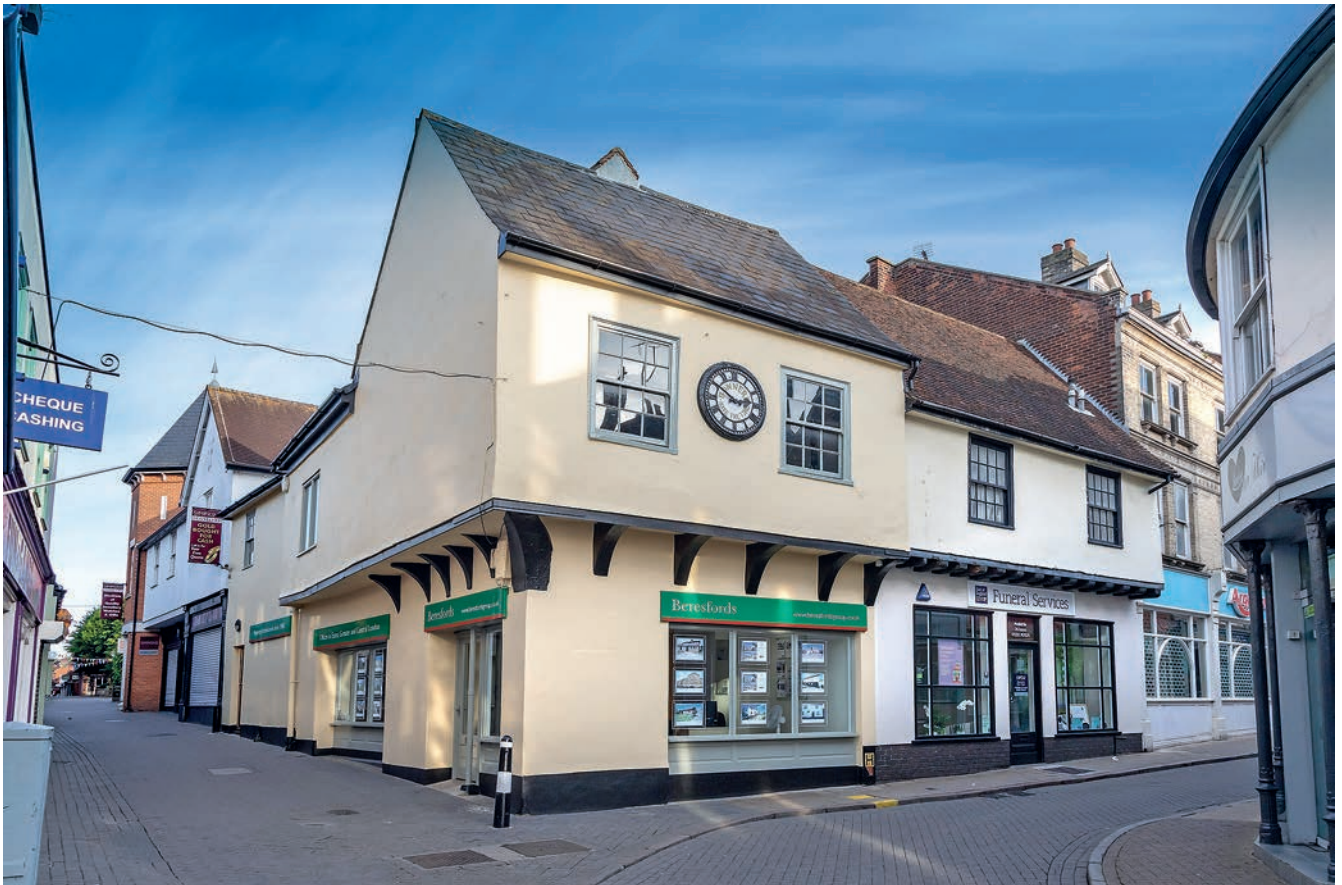
FIGURE 228: (below) 37 Long Wyre Street (corpus no. 55). The adjacent long-wall jetty building (Co-op Funeral Services, 33–5 Long Wyre Street) has not been surveyed
