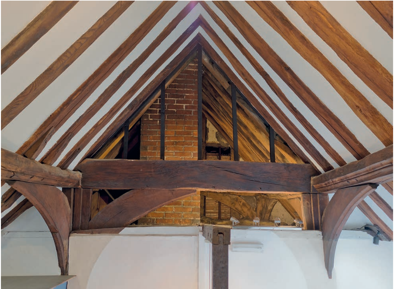
FIGURE 352: View of the roof of Part A showing the queen-post roof, inside GfB, The Colchester Bookshop, 7 Trinity Street, Tymperleys (corpus no. 93). Jess Tipper
