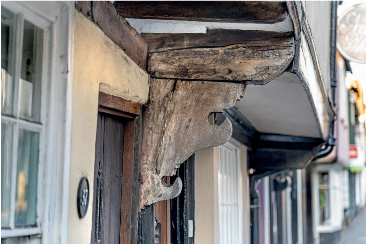
FIGURE 54: Decorative jetty bracket on 37 East Hill (corpus no. 11)
