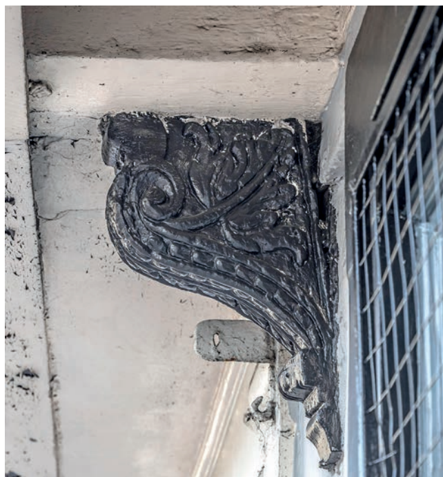
FIGURE 330: (above) Decorative jetty bracket on 4a Scheregate and horned jetty bracket (right) on 28a St John's Street (corpus no. 88). Jess Tipper
