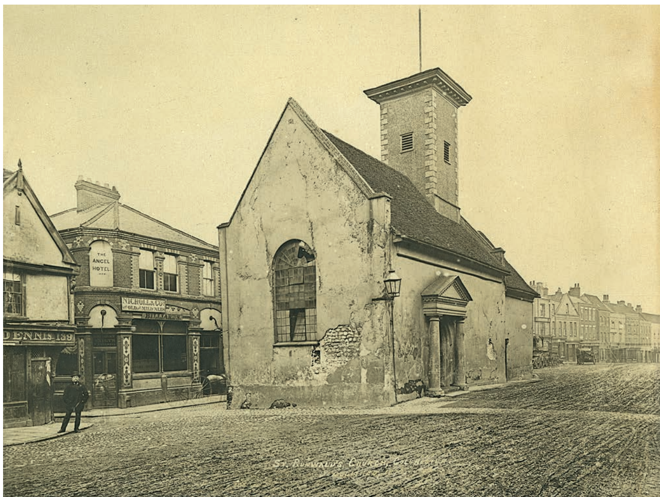
FIGURE 183: St Runwald's Church, High Street, prior to demolition in 1887. The 'Green Man' dragon post can be seen on the corner building (corpus no. 43), left, demolished for Belcher's Town Hall in 1898. Courtesy of Colchester and Ipswich Museums'
