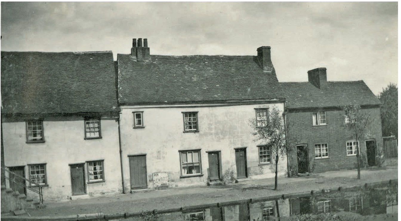
FIGURE 299: Riverside Cottages, North Station Road (corpus no. 78), taken in 1930 by George Drummond Lovell. Courtesy of Colchester and Ipswich Museums
