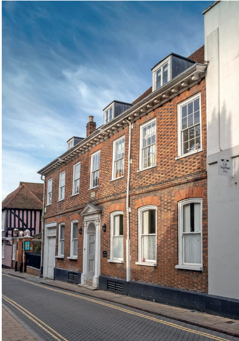
FIGURE 342: 6 Trinity Street (corpus no. 92), with decorative brick façade from the 18th century
