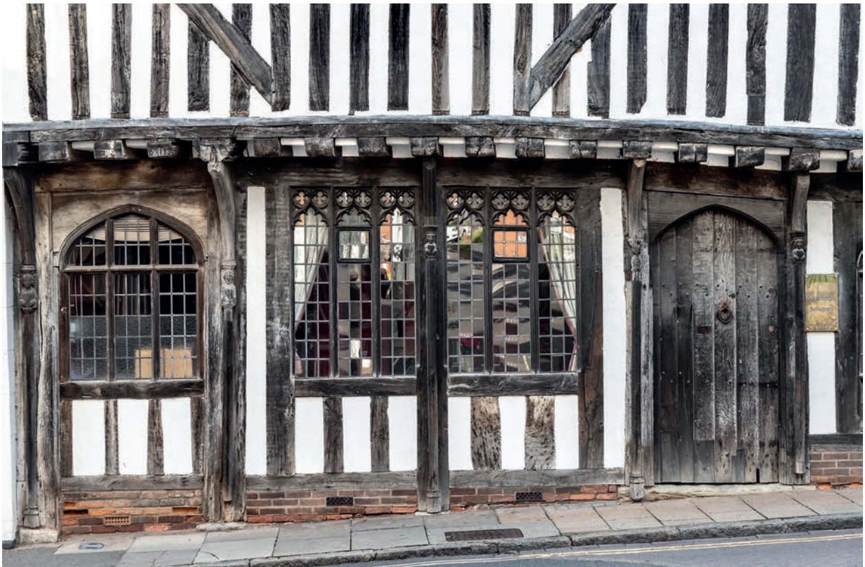
FIGURE 376: Detail of the front elevation of 3–6 West Stockwell Street (corpus no. 98). The mullion window with a traceried head was inserted during the restoration. The window on the north (left) side was originally a doorway with a flat-roofed merchant's door head (porch). Notice the carved angels each holding a shield, located at the base of each jetty bracket (and top of the pilasters), most of which are early 20th-century copies. The angel motif seems to have been popular with 15th-century merchants
