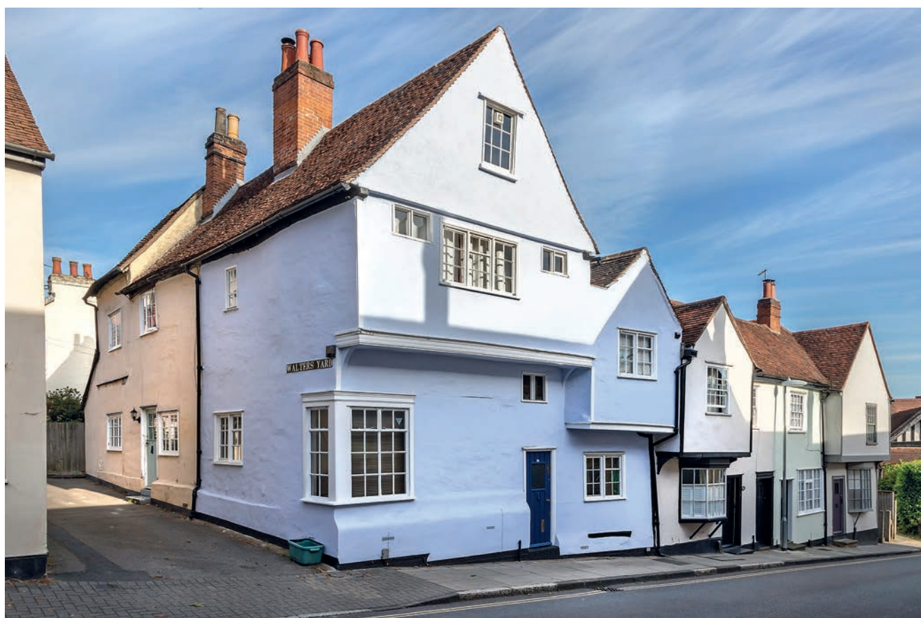
FIGURE 409: West Stockwell Street (corpus no. 106). No 56 is on the corner
