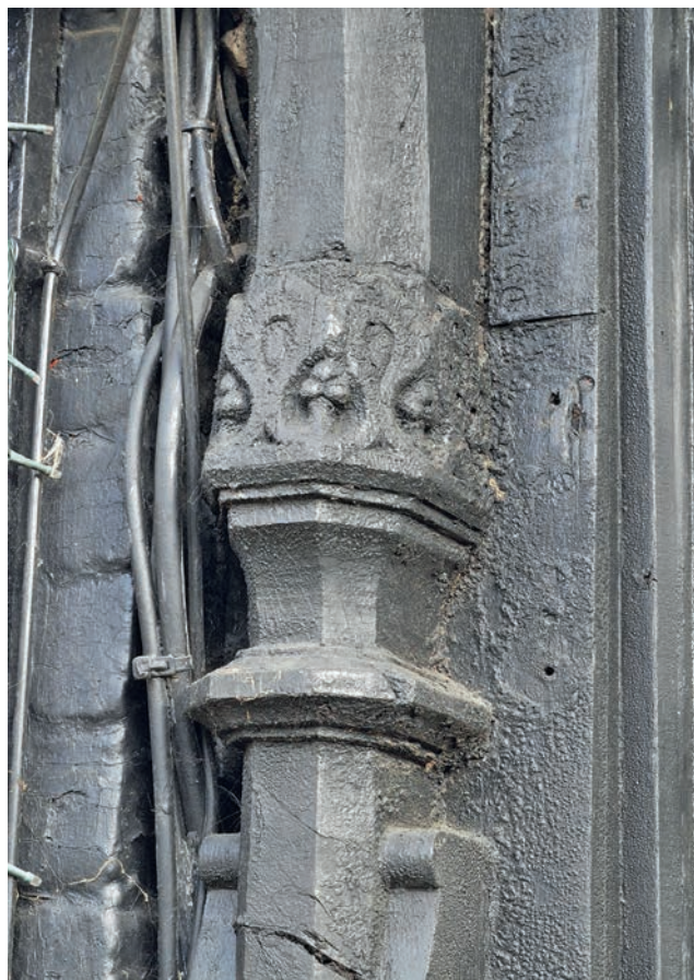
FIGURE 112: Decorative capital below jetty bracket on The Siege House, 73–5 East Street (corpus no. 24). Jess Tipper
