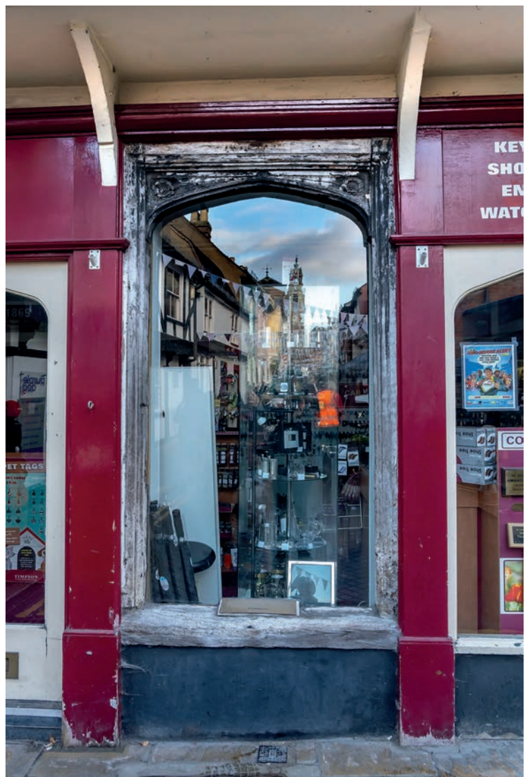
FIGURE 335: Door frame with four-centred arch head, 1–2 Sir Isaac's Walk (corpus no. 89)
