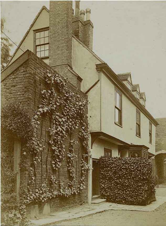
FIGURE 354: Rear extension of Tymperleys (now tea shop), 7–9 Trinity Street (corpus no. 93), taken in c.1920. Courtesy of Colchester and Ipswich Museums
