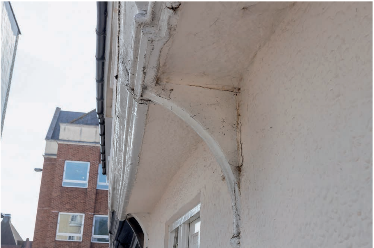
FIGURE 29: Moulded bressumer, bracket and shaft on 13 Church Street (corpus no. 3)
