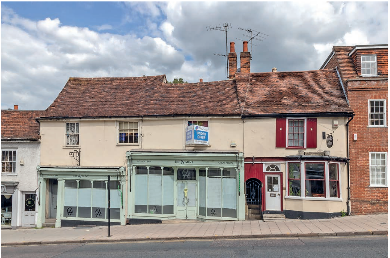
FIGURE 247: (below) 13–15 North Hill (corpus no. 63). No. 13 is on the right
