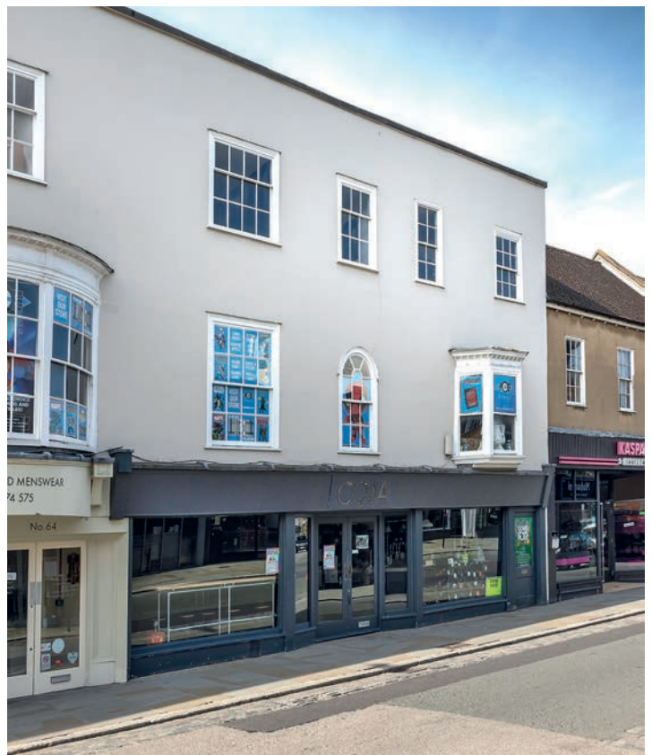
FIGURE 154: 63 High Street (corpus no. 43); the timber-frame is on the west (right) side, now with the bay window
