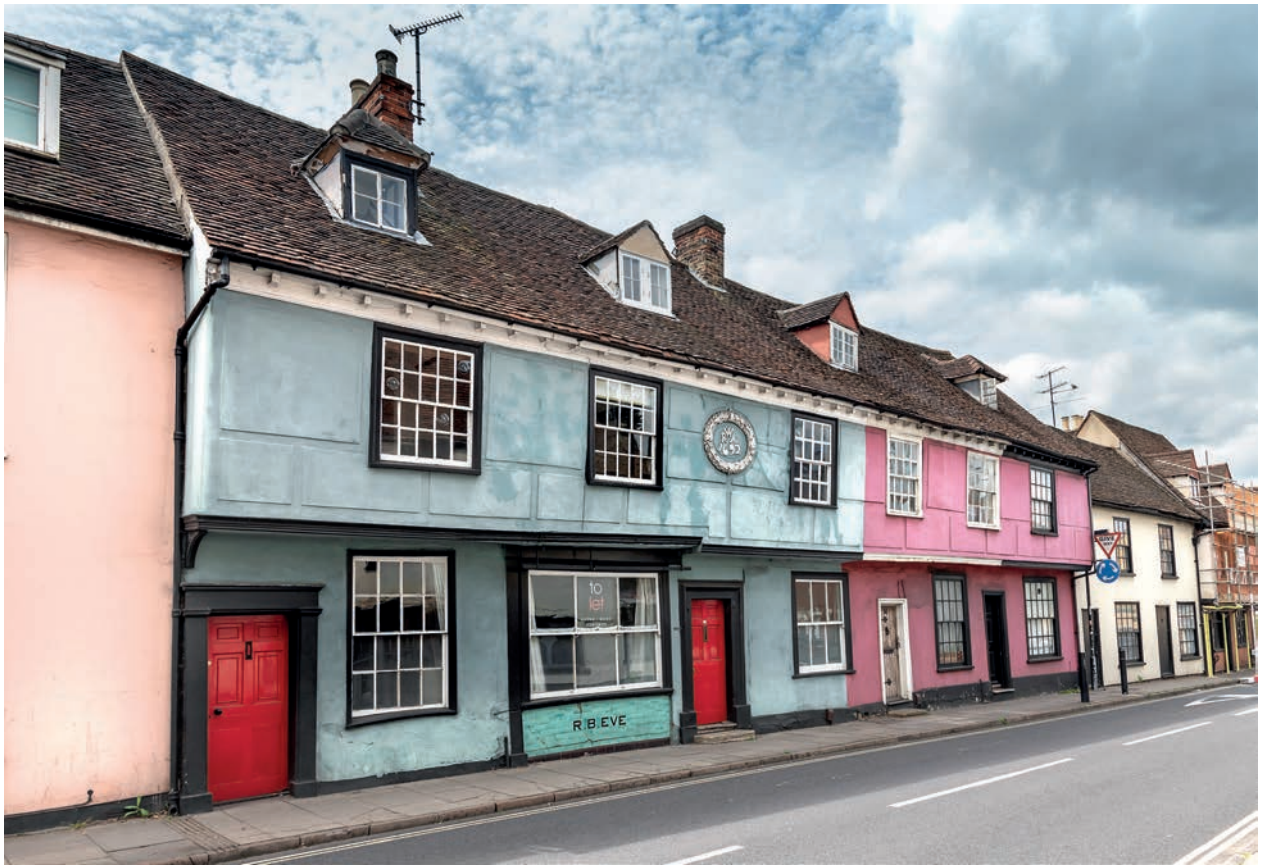
FIGURE 86: 29–33 East Street (corpus no. 20). The dormer windows with hips at either end probably date to the 1692 improvements (the others are later). No. 29 is at the right end (pink)
