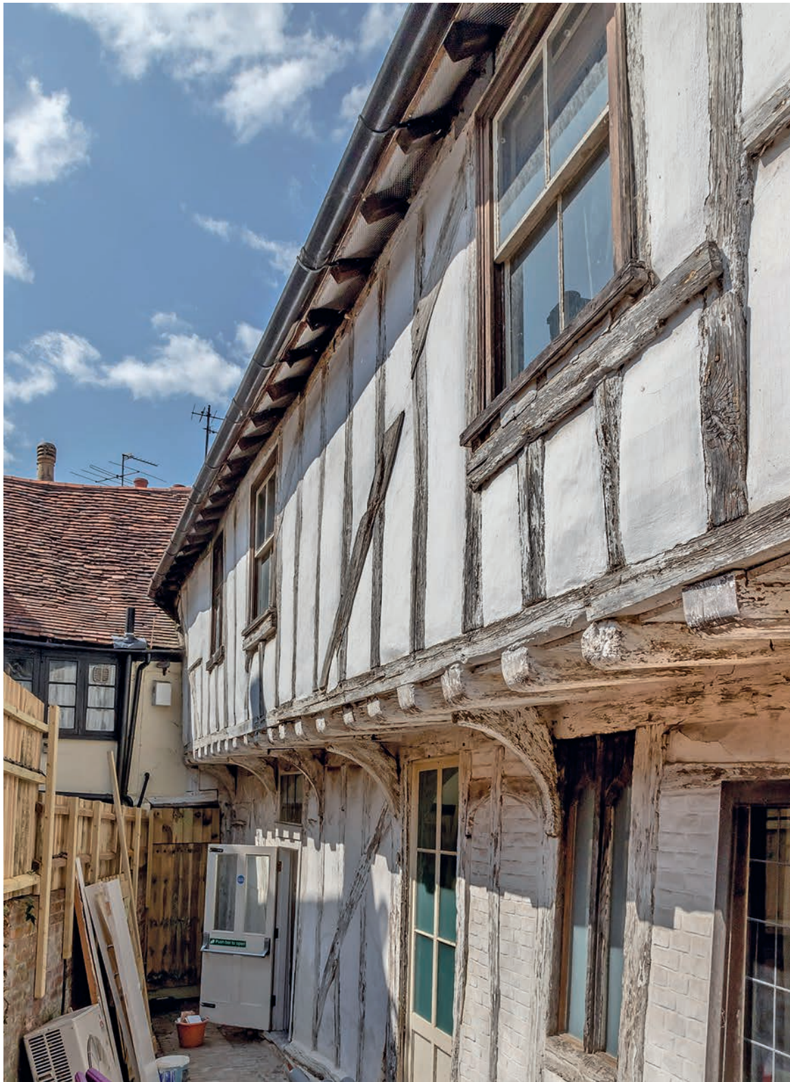
FIGURE 248: Building C (east / rear range) of 13–15 North Hill (corpus no. 63)
