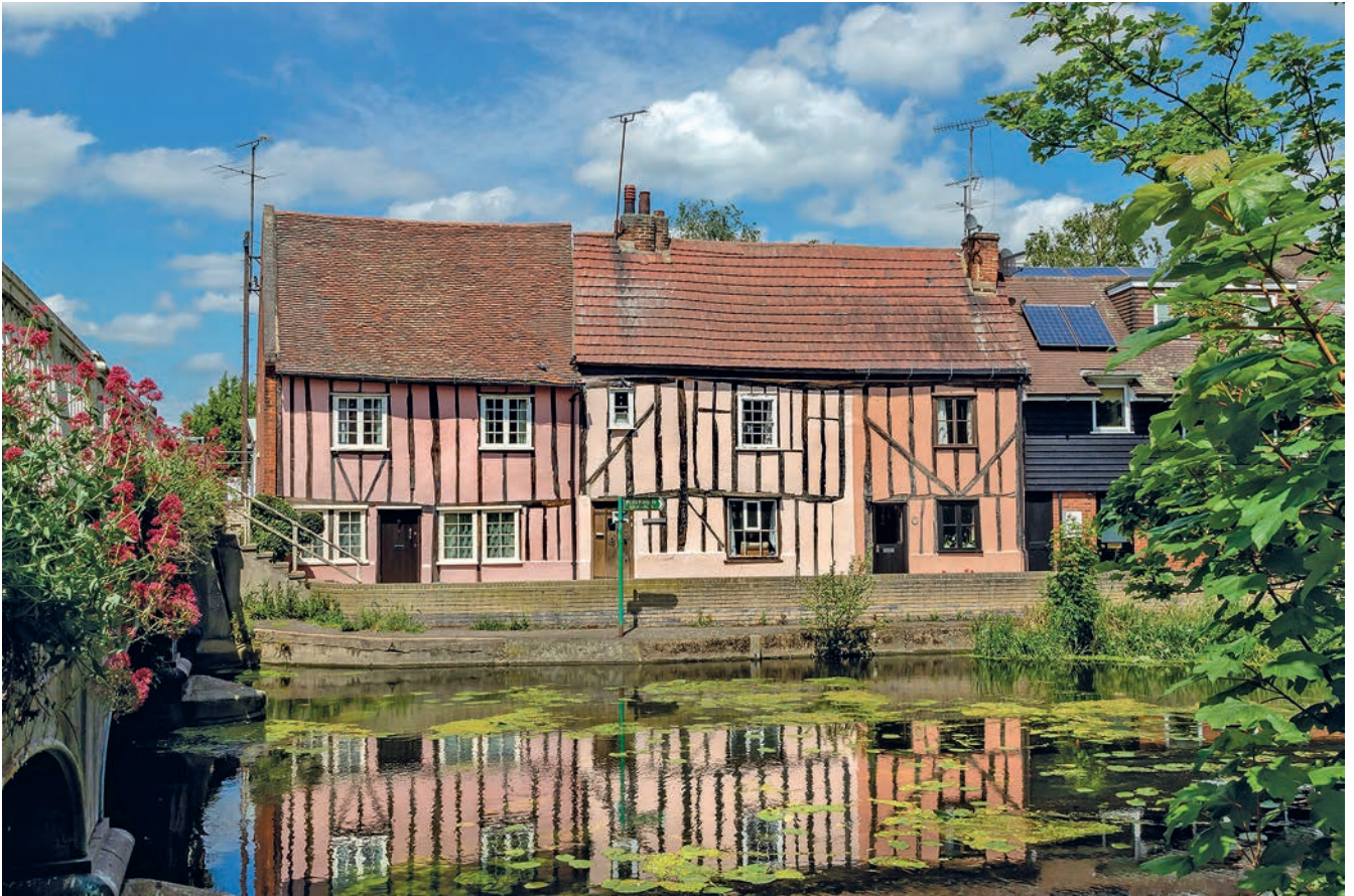
FIGURE 298: Riverside Cottages, North Station Road (corpus no. 78). 1 Riverside Walk is on the far left, closest to North Bridge
