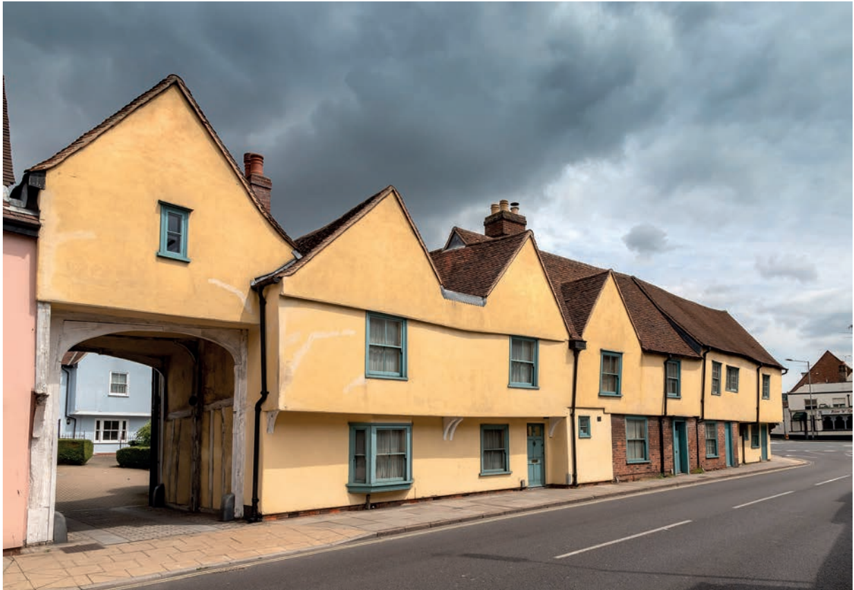
FIGURE 105: 60–5 East Street, formerly Charles Brown & Sons (from west) (corpus no. 23)
