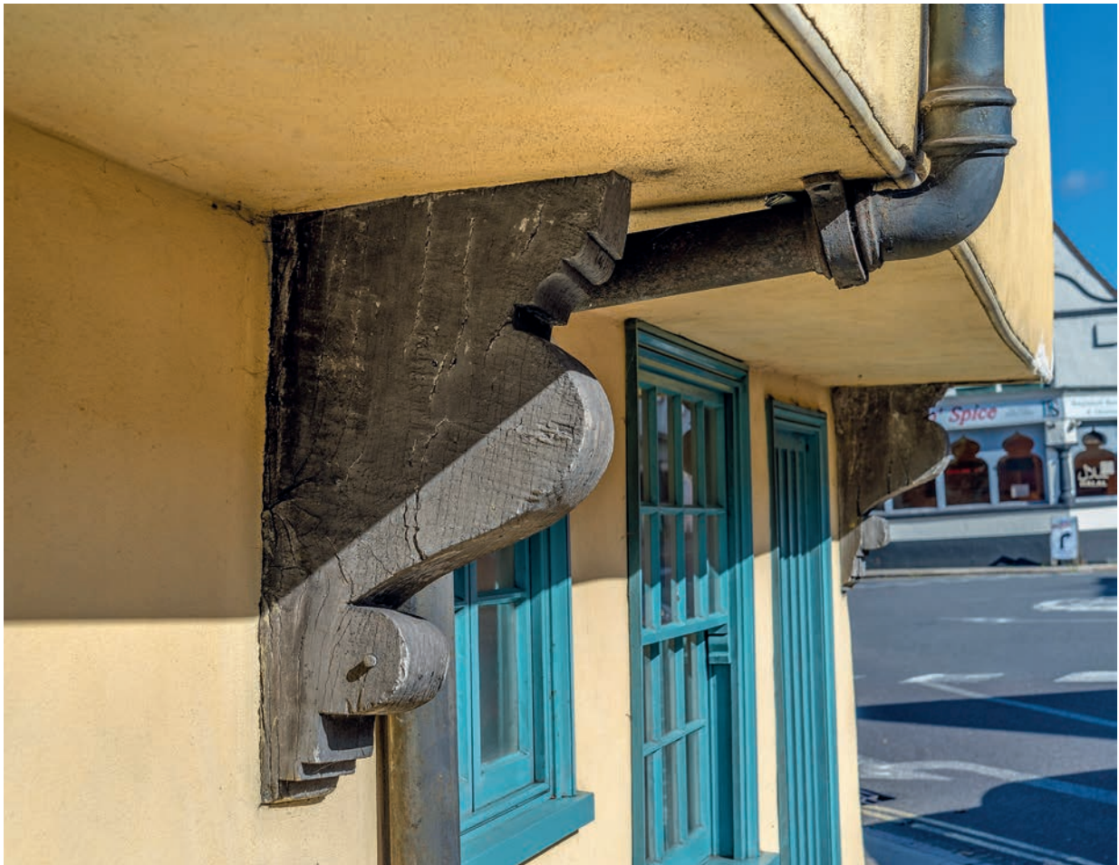
FIGURE 106: Decorative jetty bracket on 60–1 East Street (corpus no. 23), Part D
