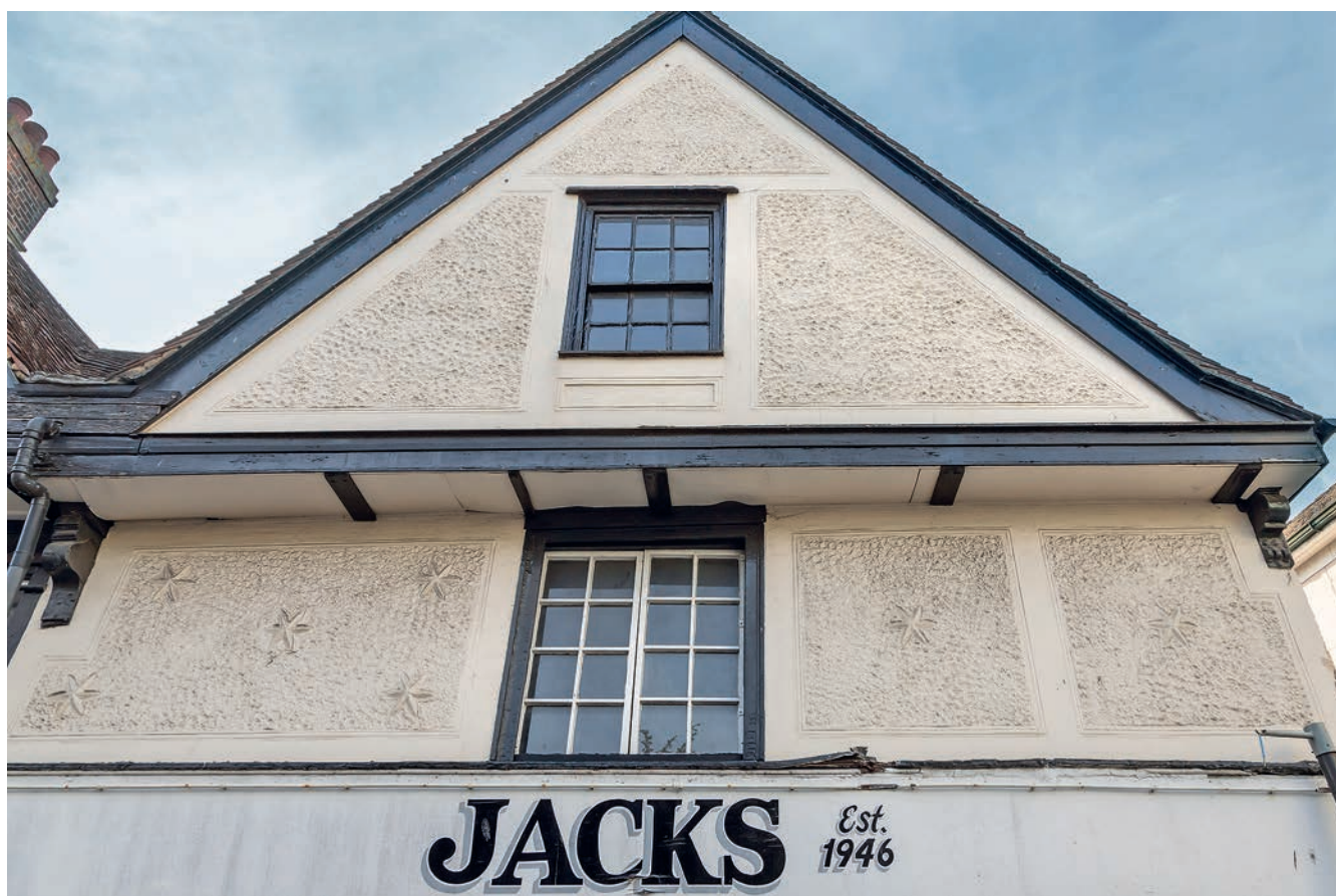
FIGURE 327: South wing of 5–6 St Nicholas Street, formerly Jacks (corpus no. 87), showing decorative eaves brackets
