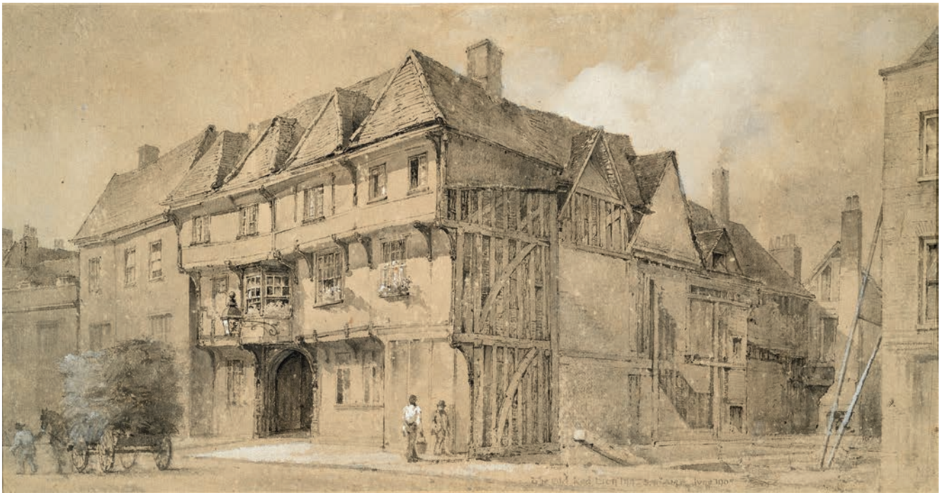
FIGURE 144: Pencil and wash drawing of The Red Lion Hotel (corpus no. 32) by Major J.E. Bale in 1905. The drawing shows the exposed west wall following the demolition of the adjacent building; notice the massive timber (presumably a cellar joist, no longer in situ ) protruding from the cellar. Courtesy of Colchester and Ipswich Museums
