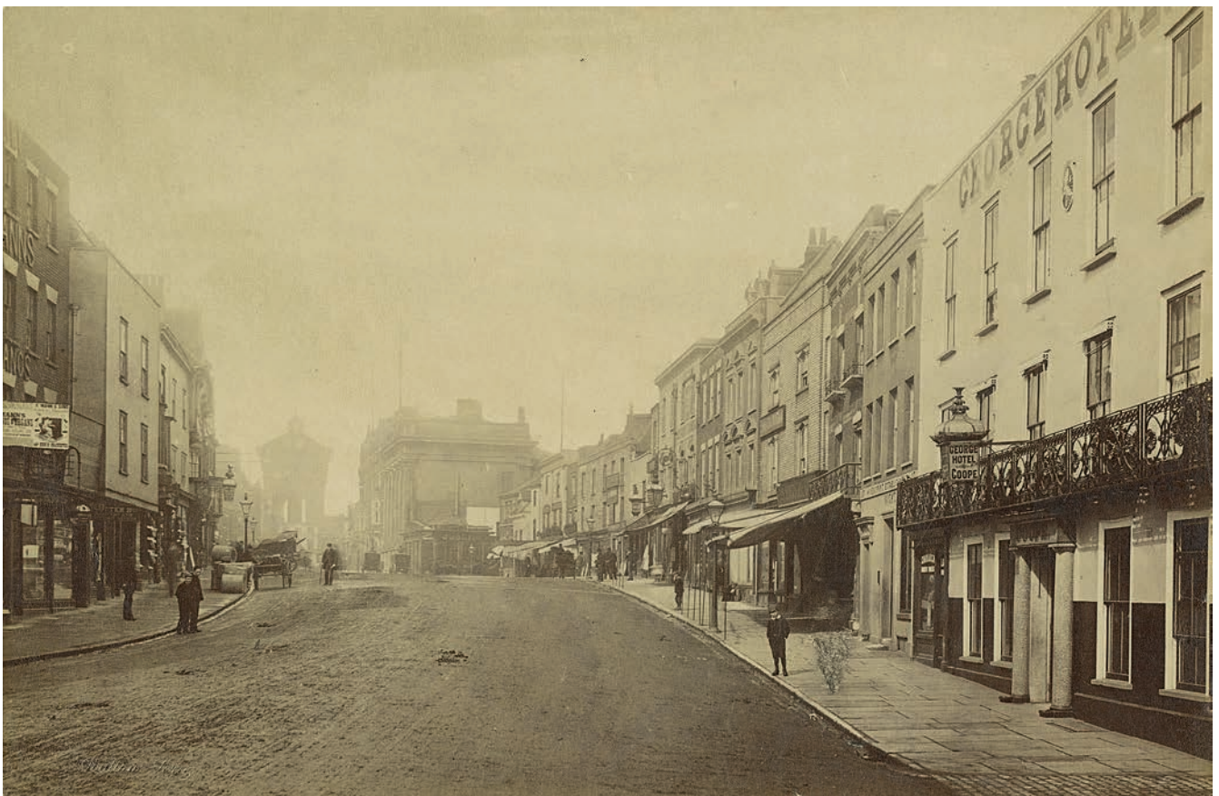
FIGURE 167: View looking west along High street, c.1890. The George Hotel (corpus no. 38) is in the right foreground. The photograph was taken before the construction of Belcher's Town Hall in 1898. Courtesy of Colchester and Ipswich Museums
