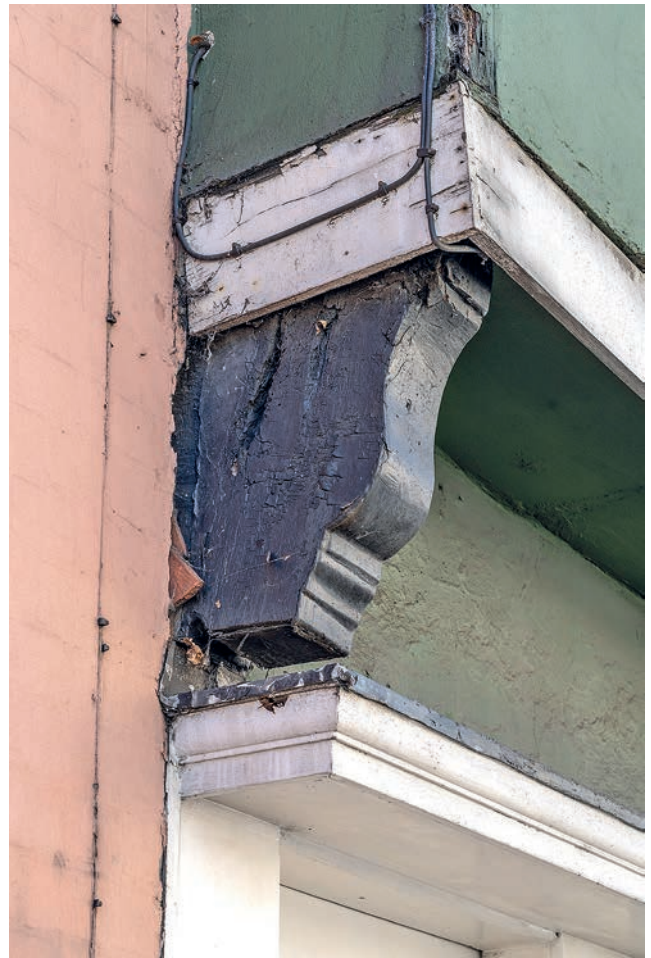
FIGURE 47: Jetty bracket on 29 East Hill (corpus no. 9)
