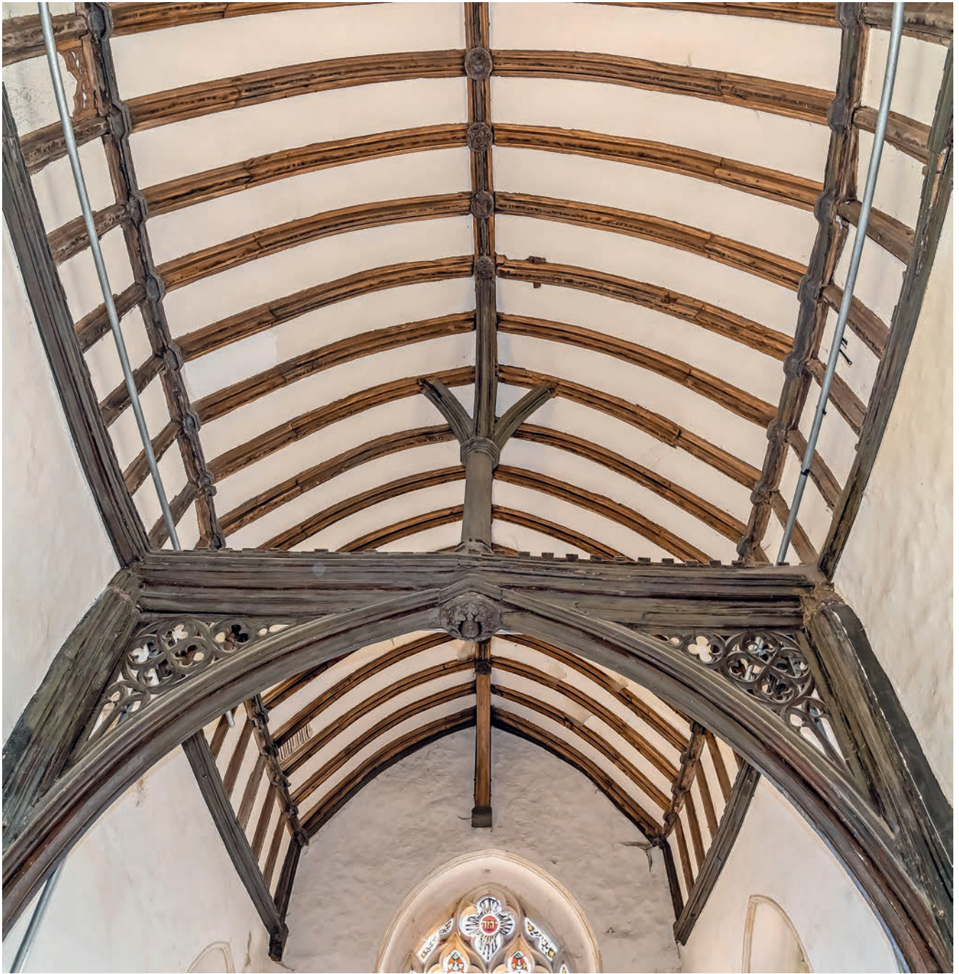
FIGURE 416: The chancel of St Martin's Church, West Stockwell Street (corpus no. 107), showing the 14th-century roof truss forming an open screen in the chancel, the arch below with traceried spandrels, octagonal crownpost with moulded four-way bracing and wagon roof with curved ribs
