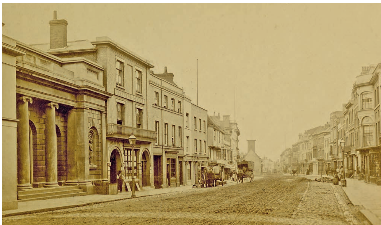
FIGURE 184: View looking west along High street, c.1870, before the demolition of St Runwald's Church in 1878. The three-storey timber-framed building of 152 High Street (corpus no. 44) is next to the horse and cart. Courtesy of Colchester and Ipswich Museums
