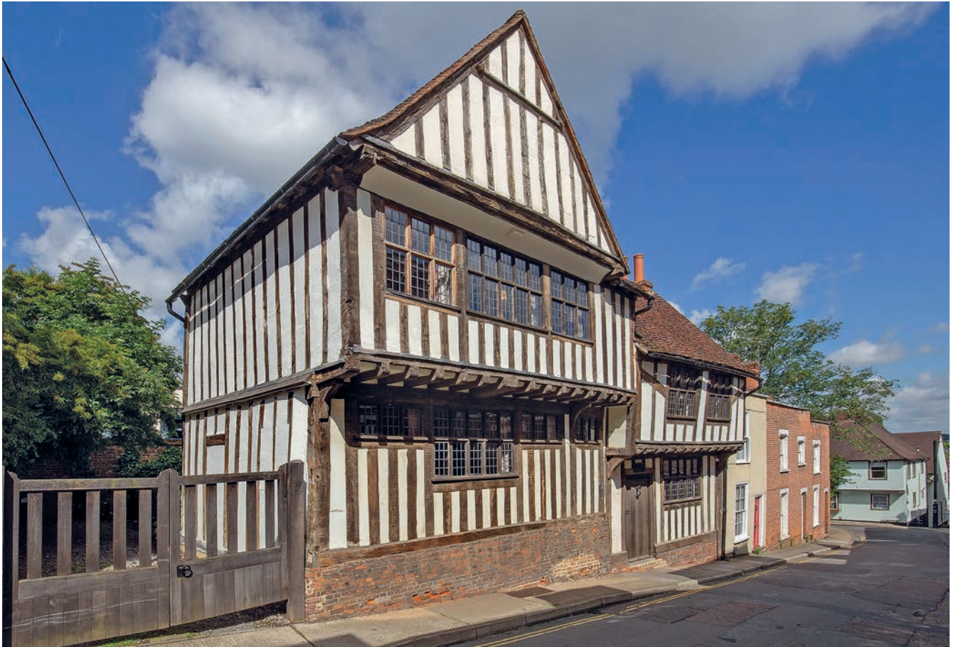
FIGURE 75 Peake's House, 30–2 East Stockwell Street (corpus no. 16). The Part A cross-wing, demolished in the 1930s, was located to the south in the area of the gates
