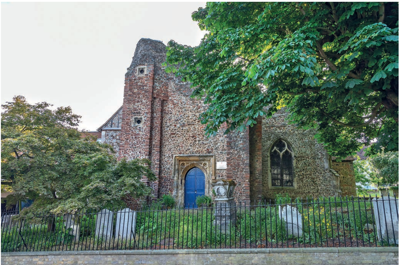
FIGURE 414: St Martin's Church, West Stockwell Street (corpus no. 107)
