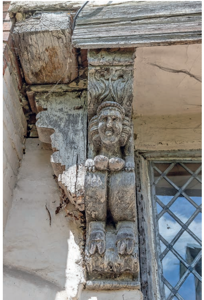
FIGURE 281: (below left and right, and opposite) 47 North Hill (corpus no. 70). Finely-carved jetty brackets on south-facing flank
