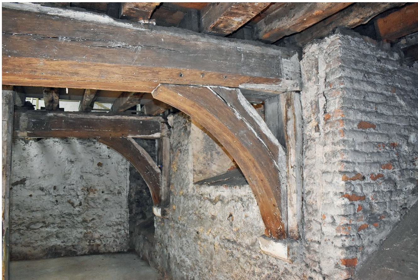
FIGURE 136: View of the cellar below Rebow House (corpus no. 31). The massive cellar joists are tree-ring dated to AD 1370–80. Courtesy of Colchester Archaeological Trust
