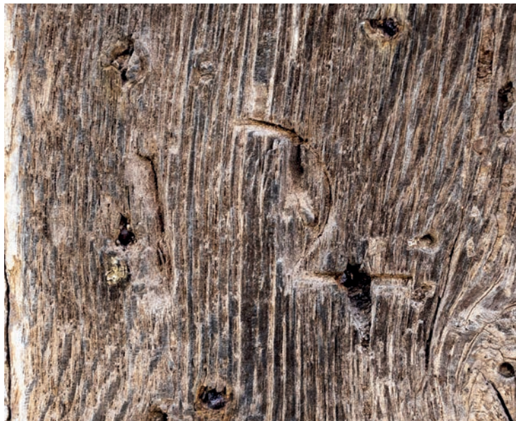
FIGURE 76: Peake's House, 30–2 East Stockwell Street (corpus no. 16). Detail of carpenter's mark on one of the Part B frontage studs using Arabic numerals (No. 12)
