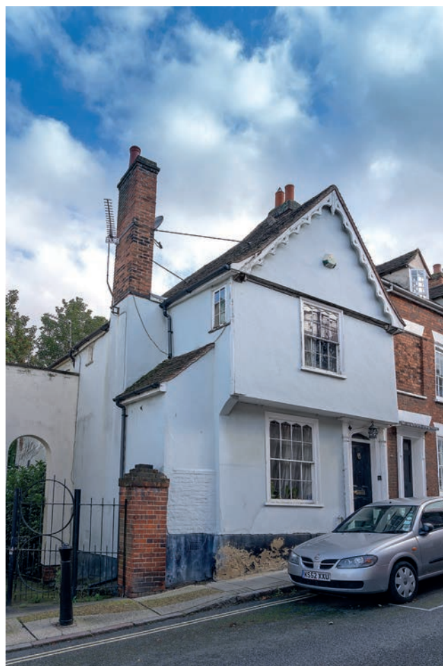
FIGURE 379: 13 West Stockwell Street (corpus no. 99). Notice the chamfered tie beam on the front elevation
