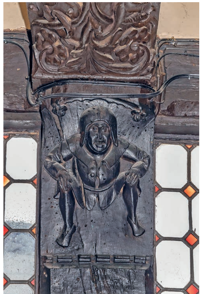
FIGURE 260: (below left and right) Two finely-carved brackets supporting the bridging joist in the rear wing of The Marquis of Granby, 24 North Hill (corpus no. 66)
