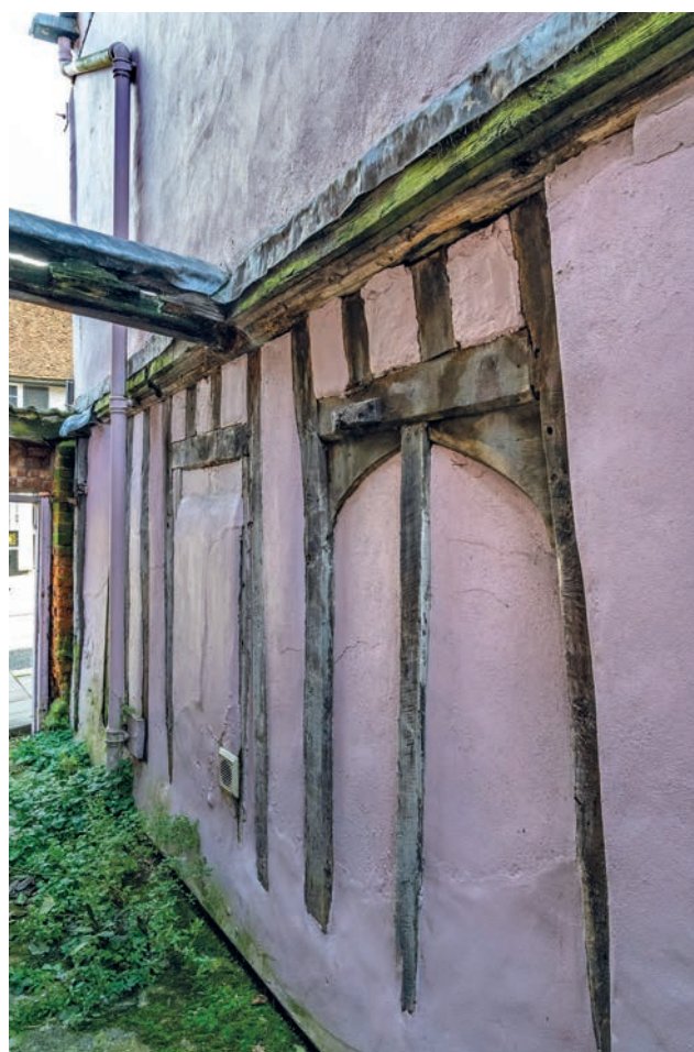
FIGURE 271: North wall of 37 North Hill (corpus no. 68) showing the remains of the two service doors
