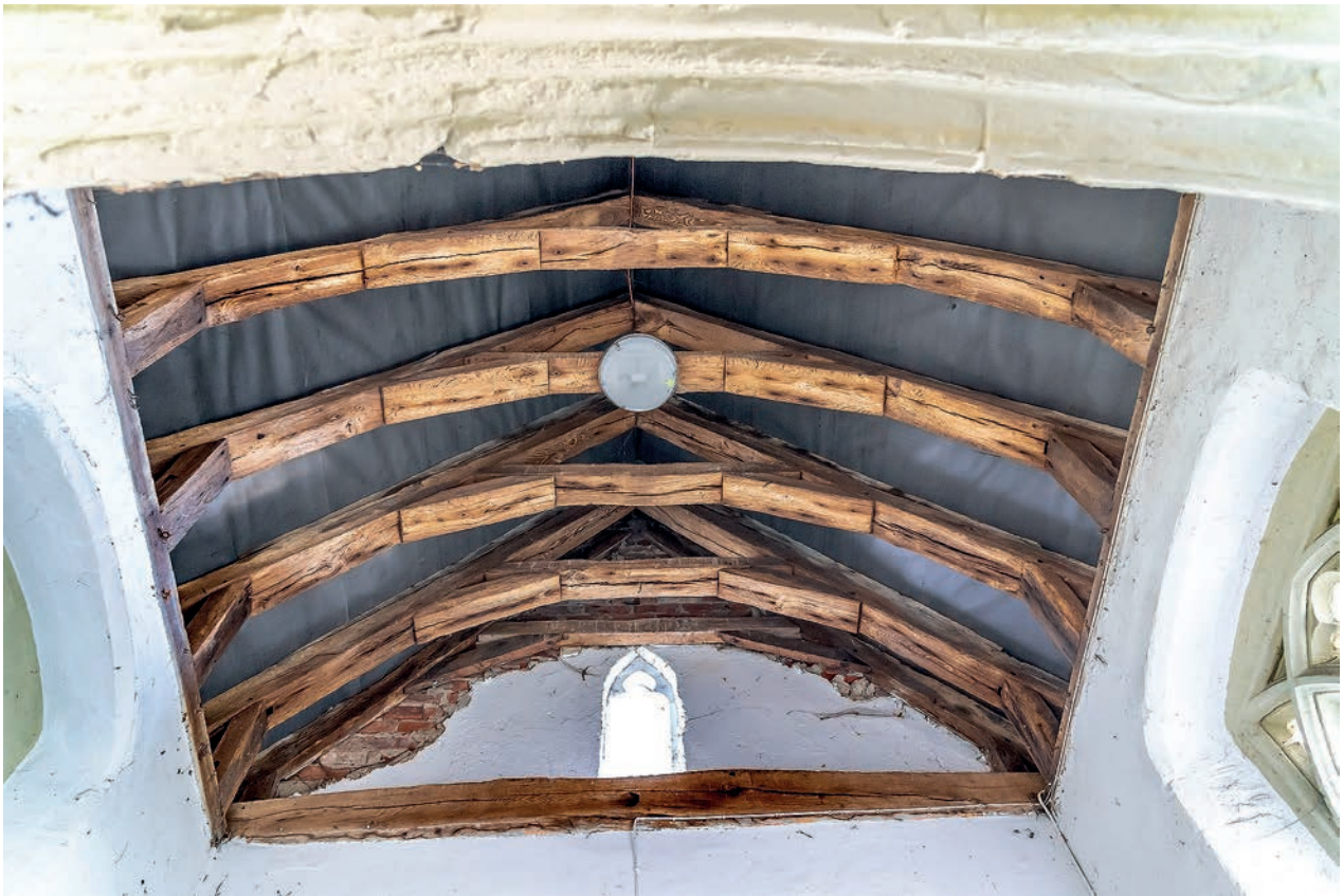
FIGURE 368: The seven-cant roof in the porch of Trinity Church, Trinity Street (corpus no. 97)
