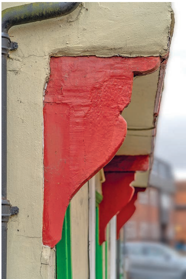
FIGURE 302: Decorative jetty bracket on 13 and 15 Northgate Street (corpus no. 79)
