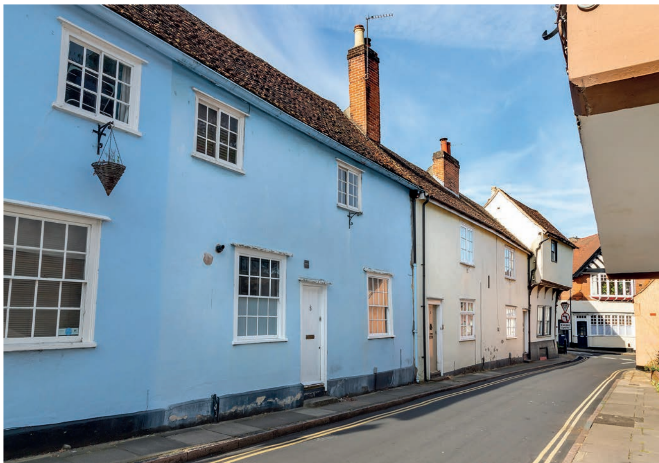
FIGURE 340: 3 and 5 Stockwell (corpus no. 90). (The Stockwell Arms, 18 West Stockwell Street (corpus no. 101) is on the right, on corner of the street)
