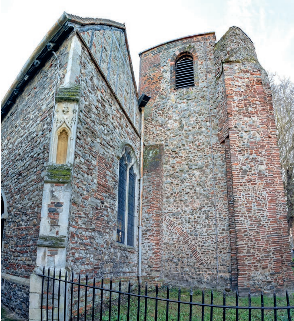
FIGURE 415: West end of St Martin's Church, West Stockwell Street (corpus no. 107), showing the north elevation of the tower and west elevation of the north aisle. The corner of the early 12th-century north aisle, formed in Roman brick, is preserved in the extended wall of the 14th-century aisle. A relieving arch, also in Roman brick, is visible at the base of the late 14th-century tower
