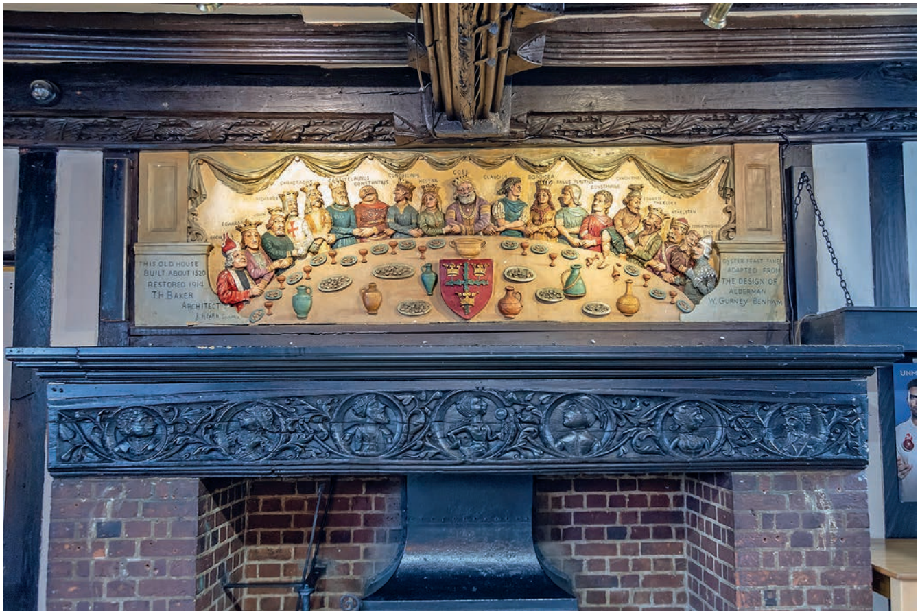
FIGURE 261: Elaborately carved ceiling joist and (re-used) beam over the early 20th-century fireplace, and the bas relief designed by Gurney Benham of people connected with the town's history at the Oyster Feast, in the rear wing of The Marquis of Granby, 24 North Hill (corpus no. 66)
