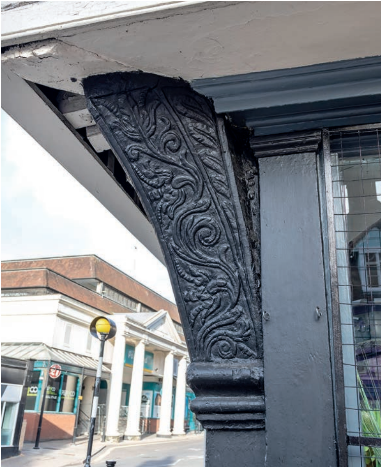
FIGURE 331: Decorative dragon post on 4a Scheregate (corpus no. 88)
