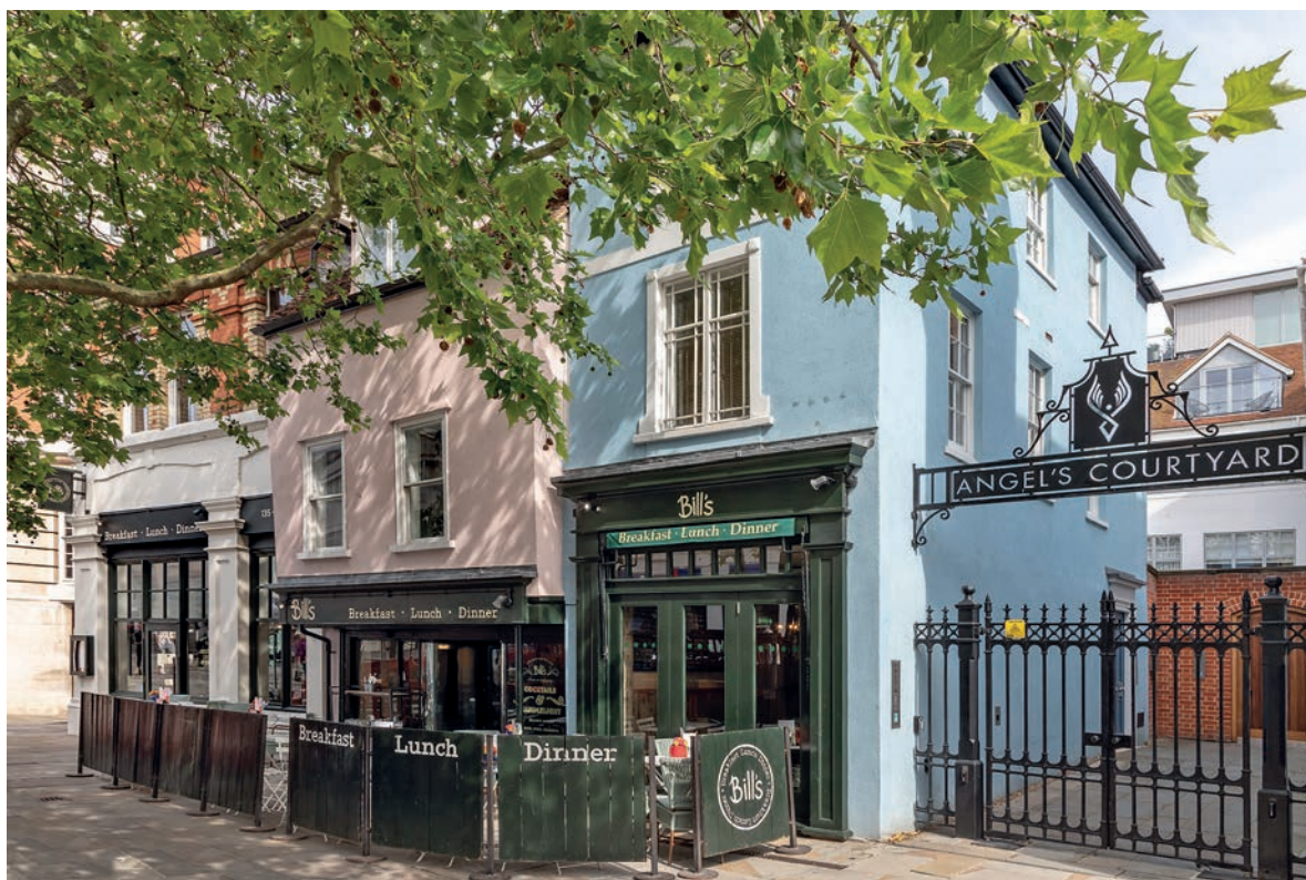
FIGURE 179: 136 High Street (corpus no. 42). No. 136 is left of centre (pink)
